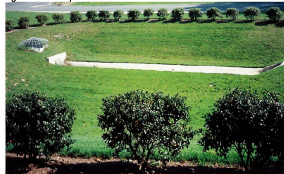
Figure A.3 Example of a Detention basin
