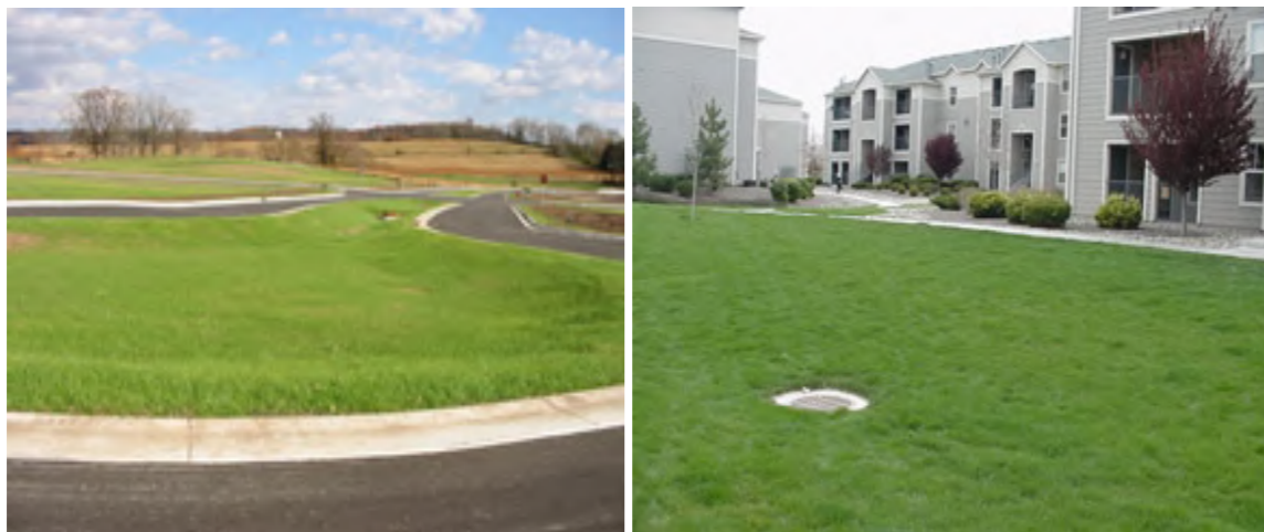
Figure A.11 Infiltration Basin
