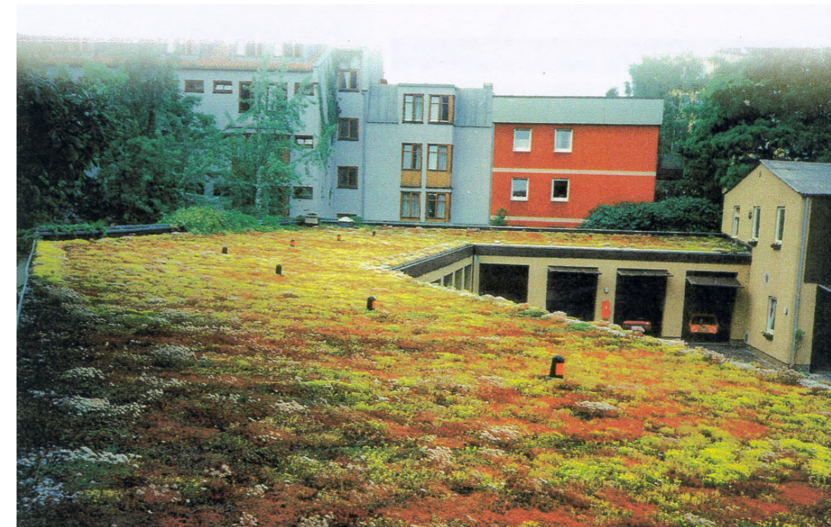
Figure A.19 Extensive Greenroof system
