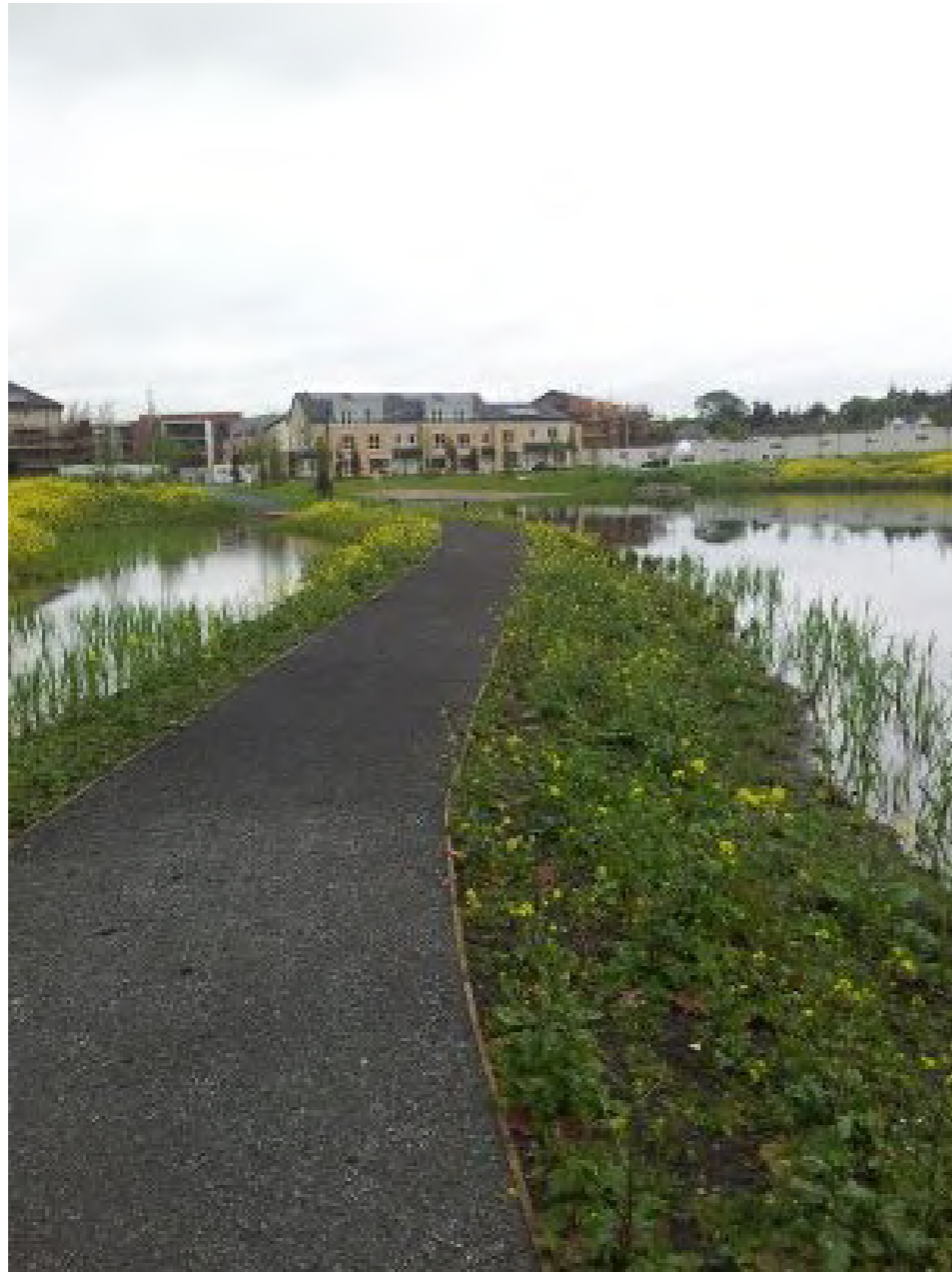
Figure A.8 Stormwater Wetland
