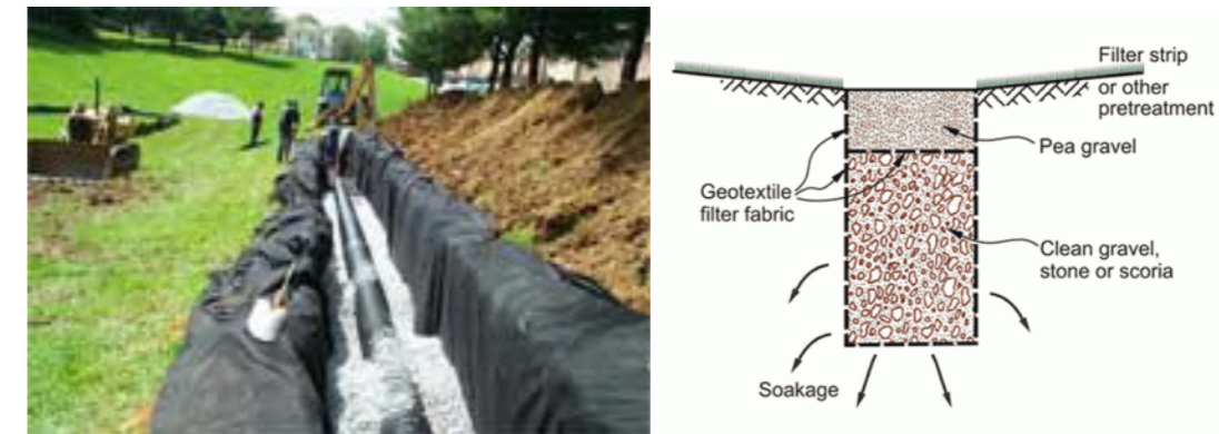
Figure A.12 Infiltration Trench
