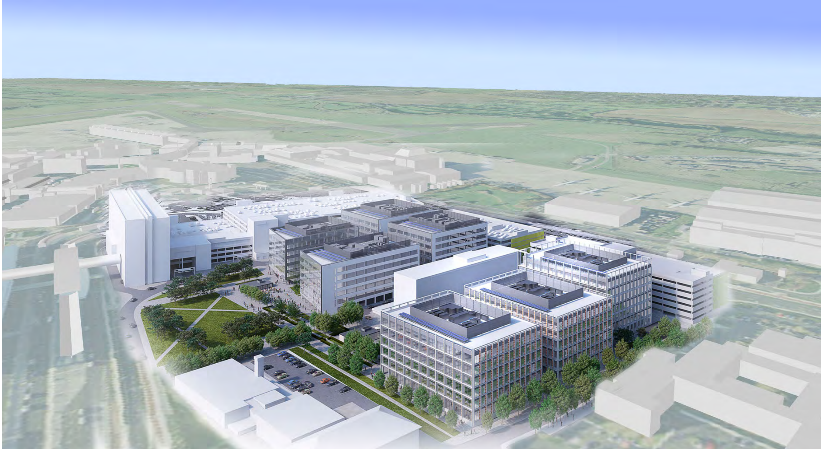
Aerial View from Southwest
