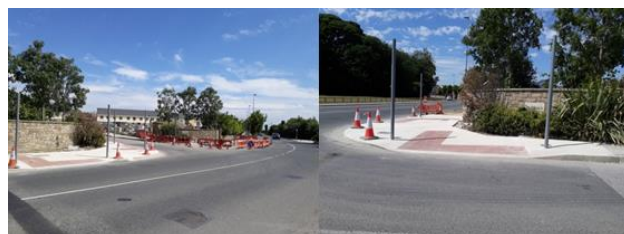
Cappagh / Heathfield traffic signals junction
