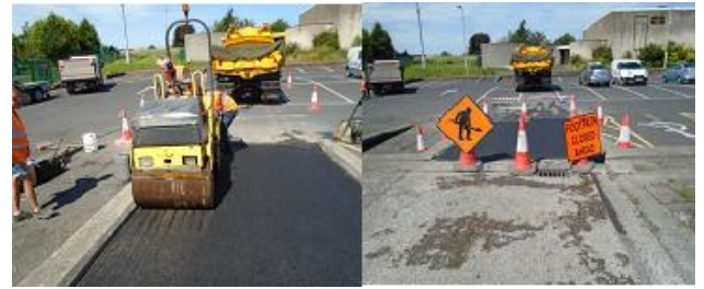
Installation of a ramp at Corduff Shops/Church for disabled access.
