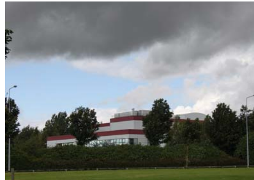
Large freestanding Industrial unit
