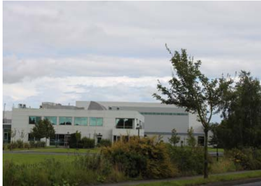
Large freestanding Industrial unit
