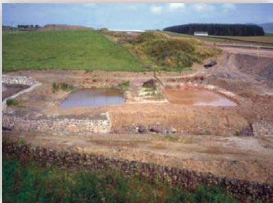
Retention Ponds, Construction Stage, M74, Scotland
