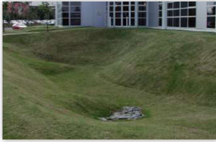
Grassed Detention Basin, South Dublin
