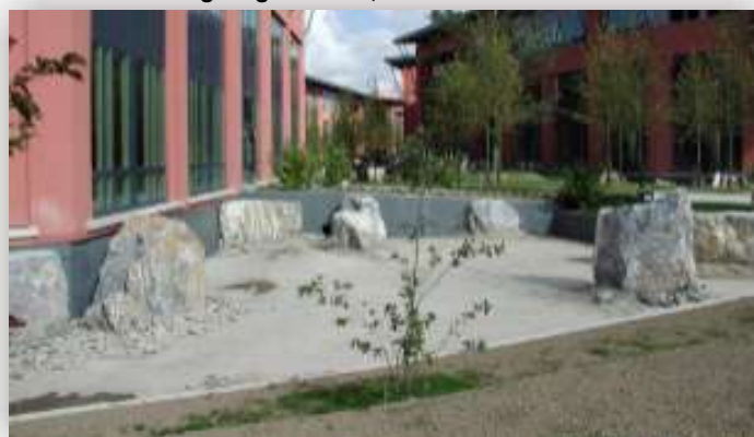
Dry Detention Basin, South Dublin
