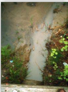
Effluent Discharge - Dry Weather Flow
