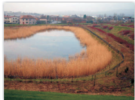
Retention Pond, Scotland
