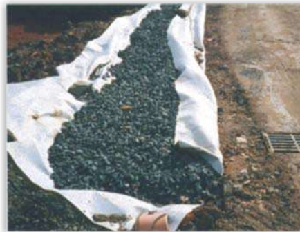
A Filter Drain under Construction
