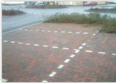
Traditional road surface drain permeable parking bays
