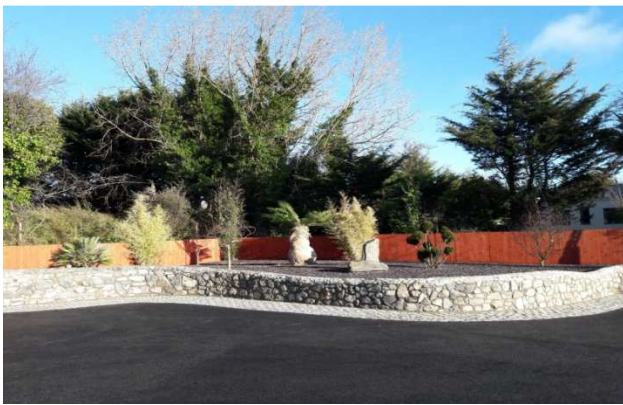
Ongoing works to the Park at The Green, Swords
