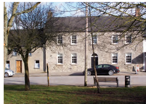
Former Barracks on Main Street
