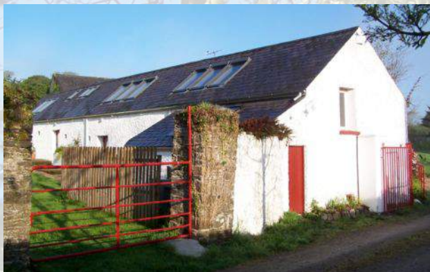
Below: Converted milking parlour with eco-friendly principles, using roof lighting to for daylight and ventilation and making it possible to retain original openings. Ballymurrin House, Wicklow,
