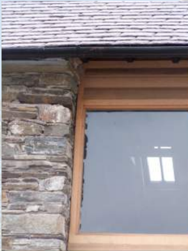
Above: Old stonework, second hand slates and new timber in Kinsale, Co Cork
