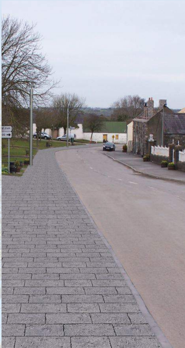
Above: Proposal to widen the pavement in the Mall is an opportunity to give precedence to pedestrian needs, whilst at the same time slowing down traffic with a narrower carriage way. In this image it has been possible to show the wirescape removed and new lights more in scale with pedestrian needs.
