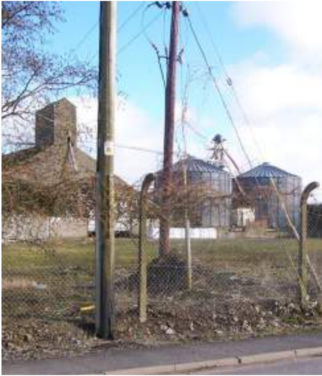
Above: Unsightly security fencing with concrete uprights and barbed wire are compromising the image of the village and its future potential. The boundary needs to be landscaped and screened.
