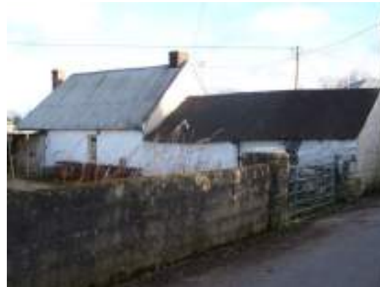
Below: Vernacular farm cottage and building close to the GAA grounds; a simple and now rare example of a small rural cottage and outbuilding.
