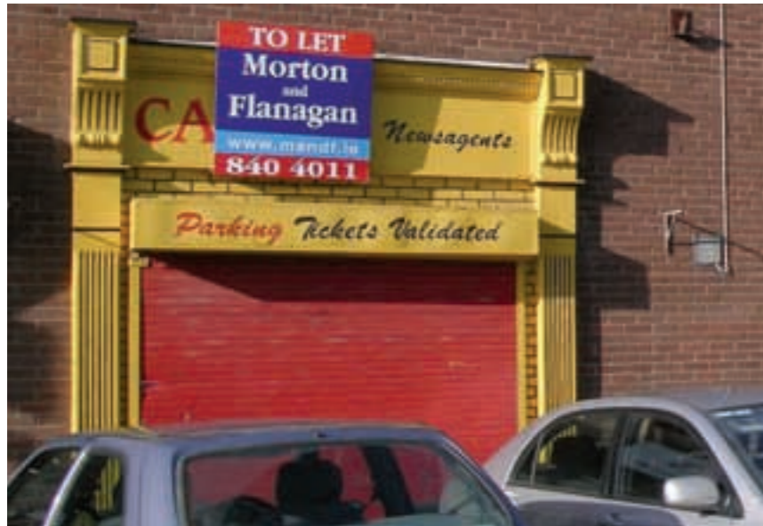
External solid shutters having a deadening effect during the day.
