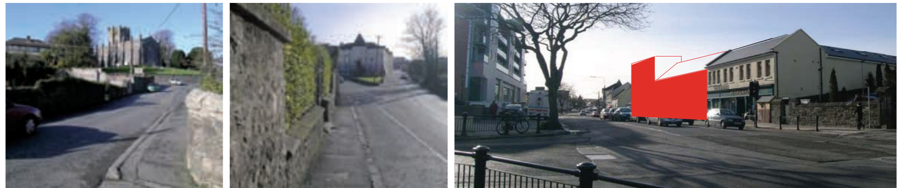
Filling out the building line
