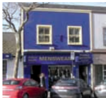
A good ratio of solid to void. The shopfronts appear vertical.
