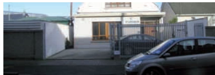
North Street: The use of high fences and walls contributes to an inactive street frontage
