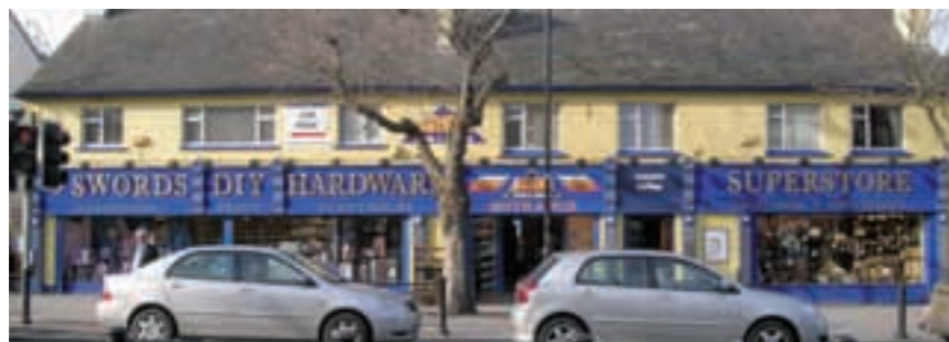
A poor ratio of solid to void. The shopfront appears too horizontal.
