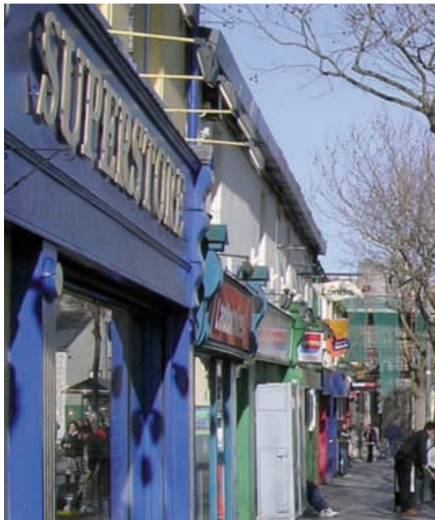
Poor quality hanging/projecting elements at various levels, serves to detract from the appearance of this group of buildings.
