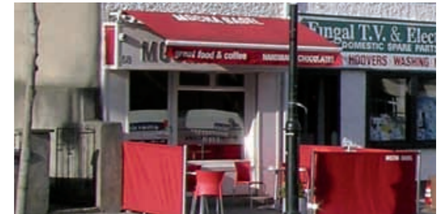
Poor design with canopy obscuring the main fascia.
