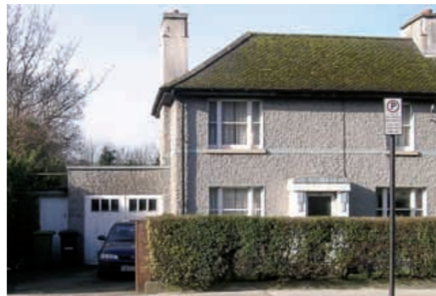
A distinctive feature is the use of hipped roofs at the end of a terrace, or on isolated properties.
