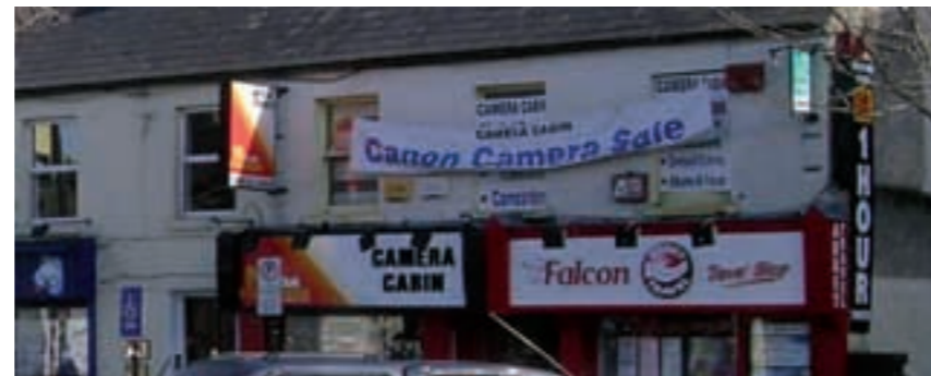
Untidy and overly busy signage is confusing. Large banner advertisements are harmful to the appearance of the traditional buildings.
