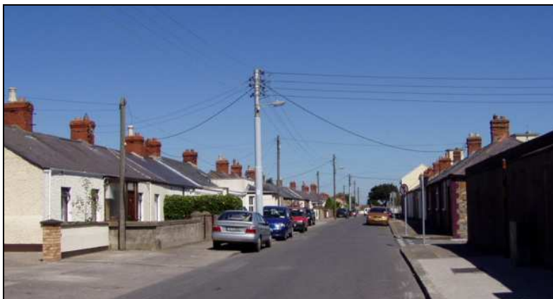
Fig. 12 College Street, looking northwards
