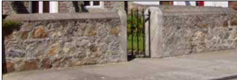
Fig. 13 Boundary wall and gate on College Street
