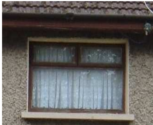
Fig. 18 House Type 2 & 3C windows -St. Sylvester's Villas
