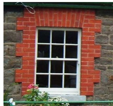
Fig. 16 House Type 1A Windows - Parnell Cottages
