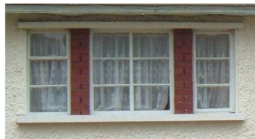
Fig. 24 House Type 3B windows
