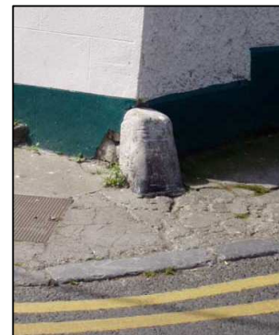
Fig. 4 Limestone Kerbing & Jostle Stone
