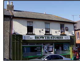
Fig. 18 No. 16 Main St before renovation
