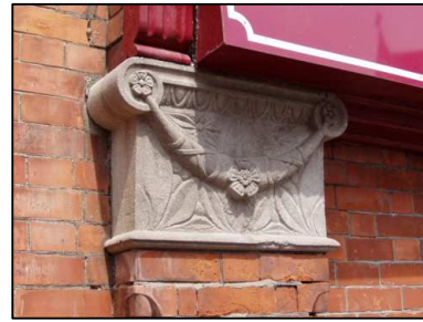
Fig. 11 Pilaster detail of No. 15 Main St
