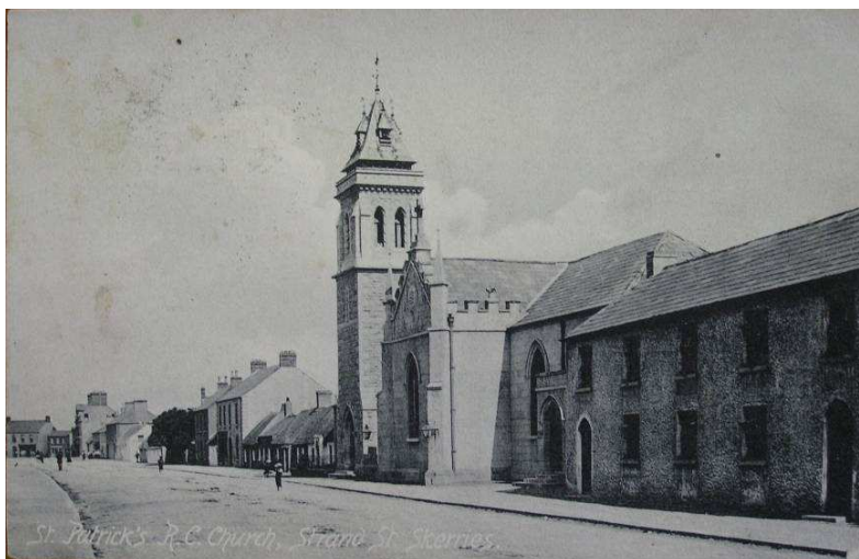
Fig 23. Church Street in an historic photograph looking north with the 1830s Catholic Church, 1884 belfry, and the former school in foreground.
