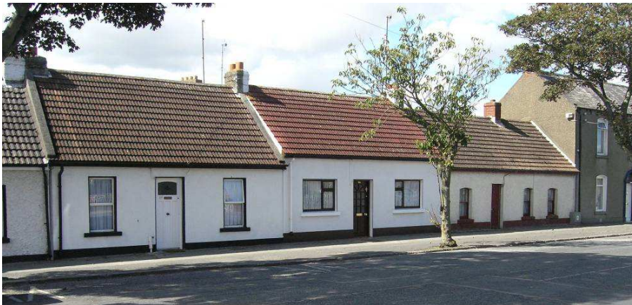
Fig. 14. Nos. 69 to 71 Strand Street: Vernacular houses compromised by tiled roofs and altered openings
