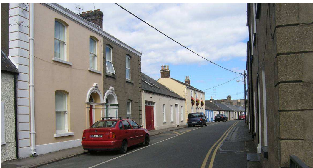
Fig. 11. Little Strand Street: Typical intermingling of single-storey vernacular and more formal two-storey houses.
