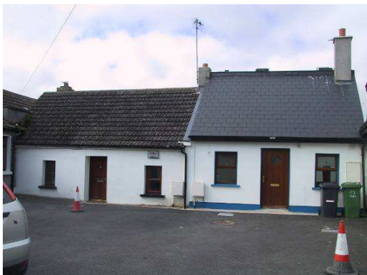
Fig 35. Altered houses at 9 and 10 The Square
