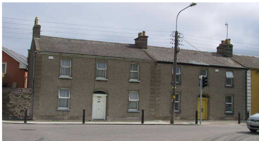
Fig. 21. Nos. 1 and 2 Church Street seen from the western part of Thomas Hand Street
