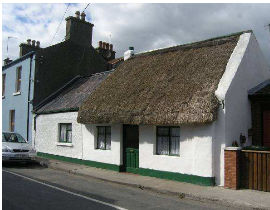
Fig 24. Vernacular thatched house at 5 Convent Lane
