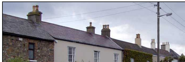
Fig. 9 Roofscape of Nos. 21 to 26 Strand Road
