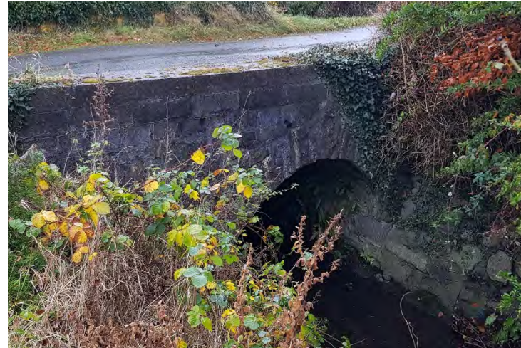
Photo 3.3.2 Arch culvert under local access road near southern boundary
