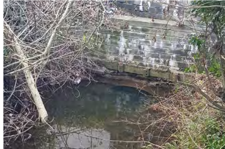
Photo 3.3.4 Downstream culvert under canal and railway
