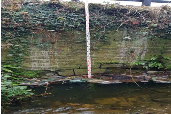
Photo 3.3.3 Upstream of canal and railway culvert
