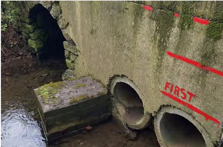
Photo 3.3.1 Three culverts under road at western boundary
