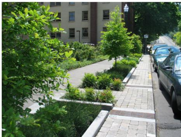
Figure 6.13 Example Roadside Bioretention Area (Portlandoregon.gov)
