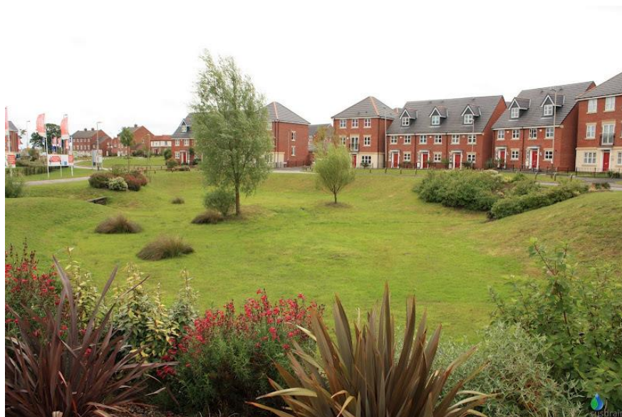
Figure 6.14 Example Detention Basin (SuDS Manual, 2015)
