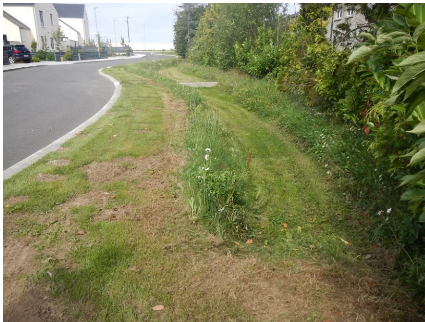
Figure 6.10 Example Roadside Swale
