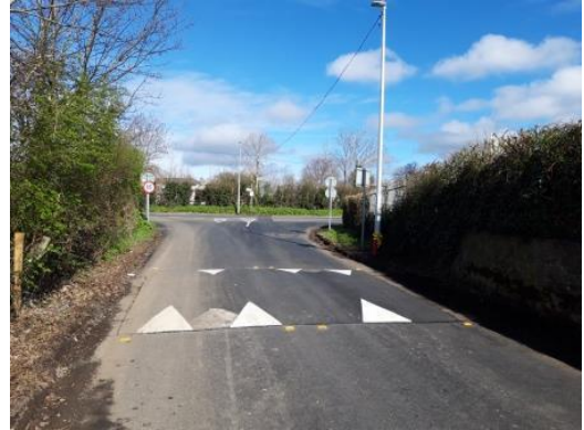
Ramps installed on Rugged Lane, Dublin 15
