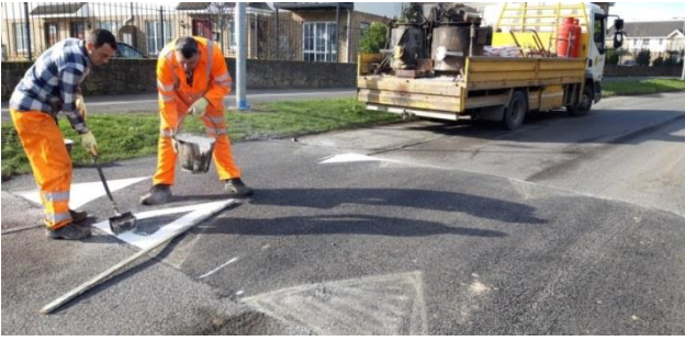
Ramp installation and road surfacing, Ministers Road, Lusk
