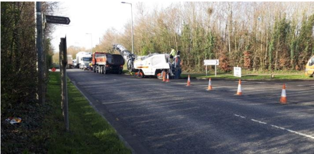
Road surfacing works, R122 to St Margaret's Village (link road)
