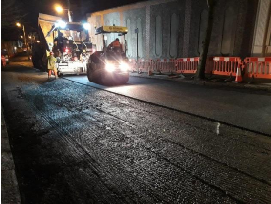
Resurfacing and relining works being undertaken in Malahide
