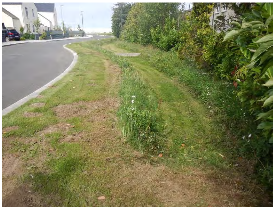
Figure 6.10 Example Roadside Swale – Emsworth Park, Kinsaley
