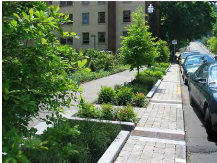
Figure 6.13 Example Roadside Bioretention Area (Portlandoregon.gov)
