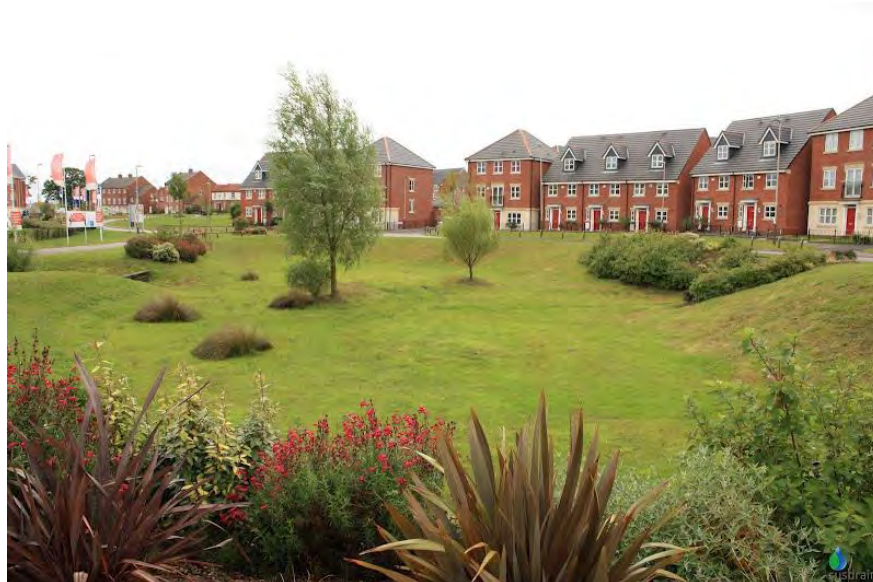
Figure 6.14 Example Detention Basin (SuDS Manual, 2015)
