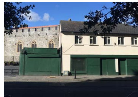
Derelict Buildings on North Street
