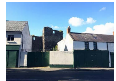
Derelict Buildings on North Street
