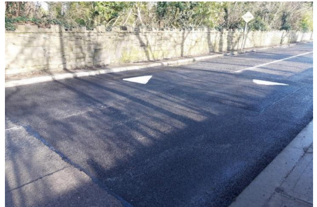
Speed Cushions repaired in Hollystown
