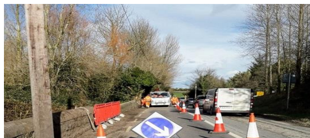
Remedial drainage works carried out on the R132 to alleviate flooding.
