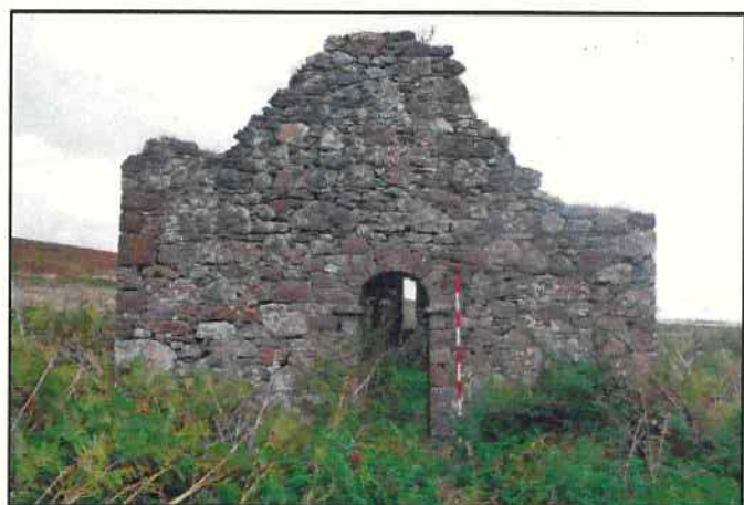
Plate 32 East gable of St Nesson's Church
