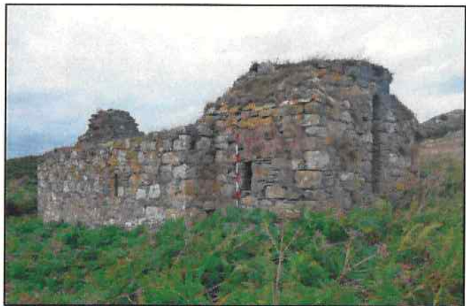
Plate 30 North walls of nave and chancel, St Nesson's Church
