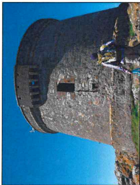
Plate 14 Martello Tower, facing north, showing raised doorway and machiolation
