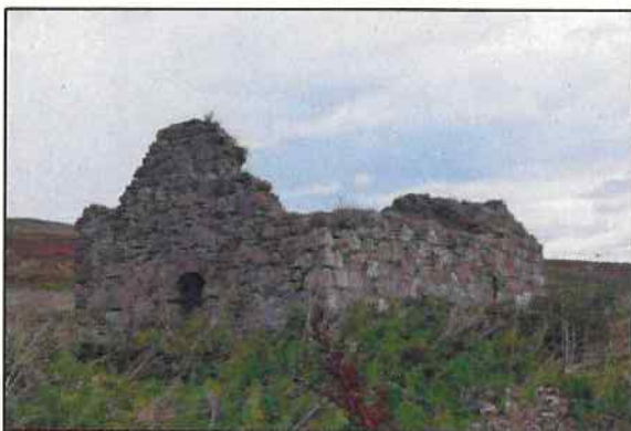
Plate 31 West gable and south wall of nave, St Nesson's Church
