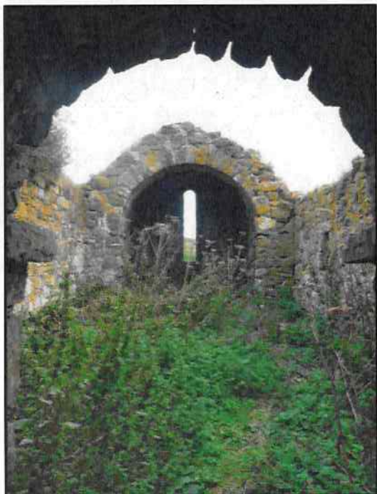
Plate 33 Interior of church: View from east doorway towards chancel
