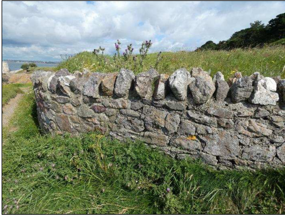
Plate 9. Rubble granite wall with rubble granite coping
