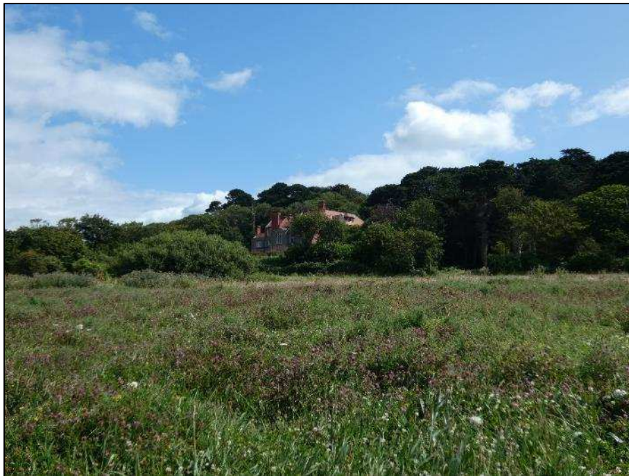
Plate 4. Sutton House and surrounding grounds
