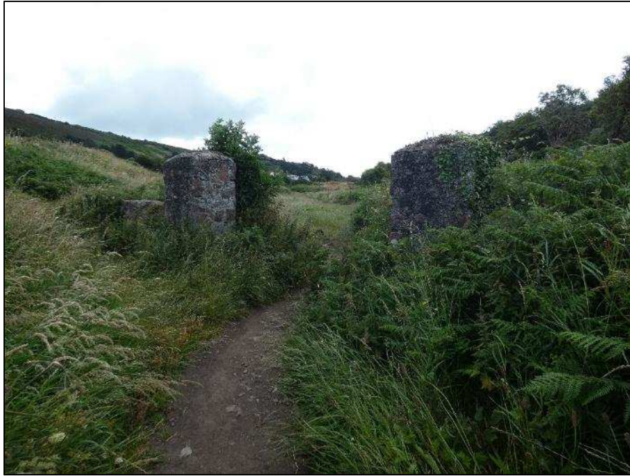
Plate 17. Piers with wall running north
