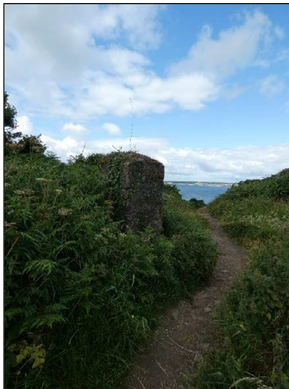
Plate 16. Rendered squared rubble granite gate pier
