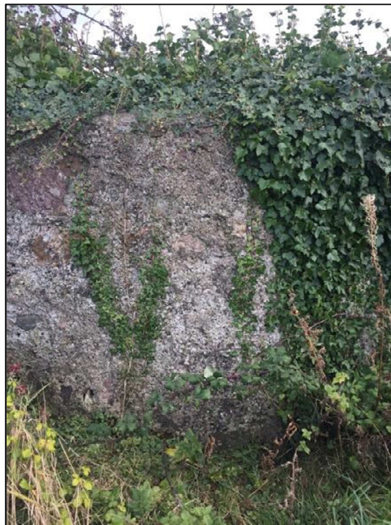
Plate 23. Southern wall of 19 th century structure
