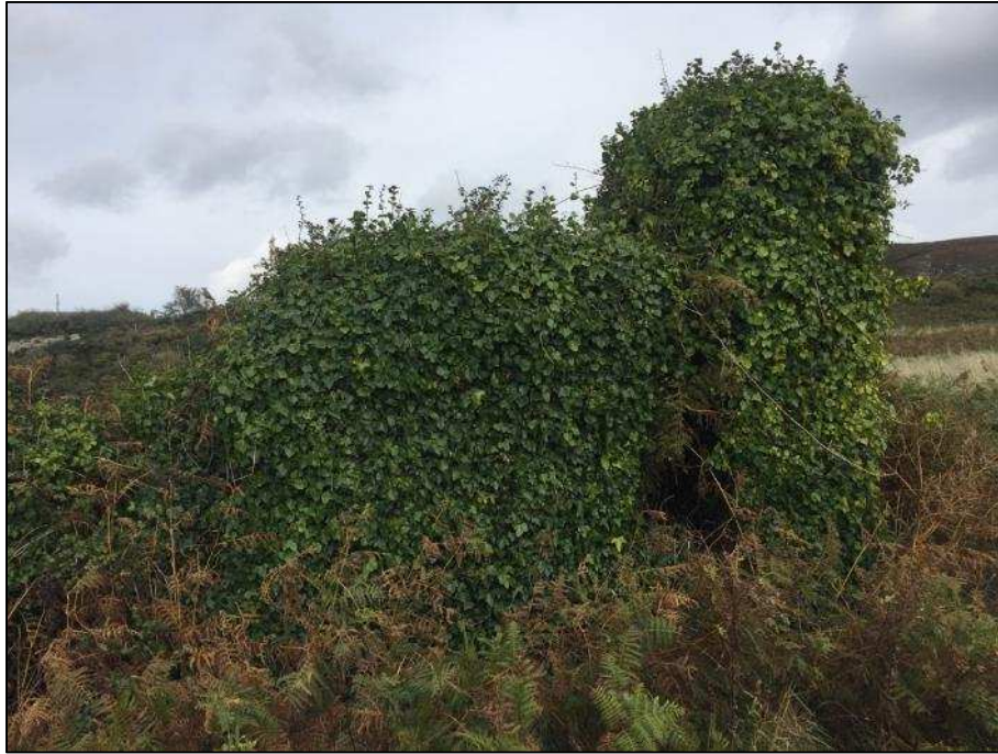
Plate 22. Eastern wall of 19 th century structure facing northwest
