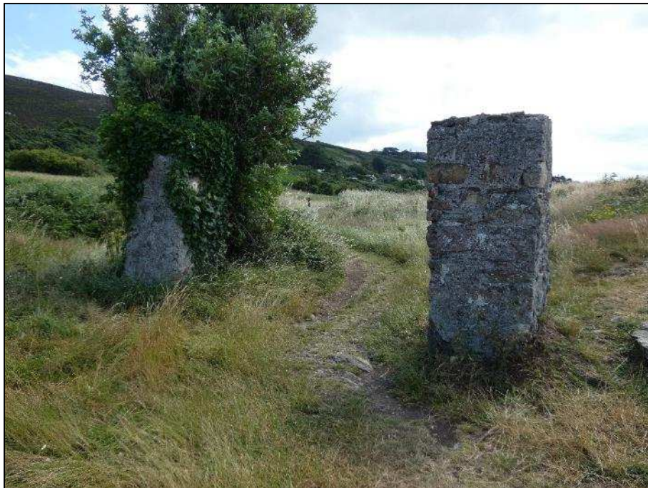
Plate 18. Pair of gate piers in the northern portion of the subject area
