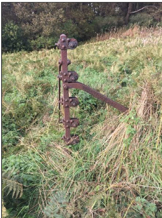
Plate 24. Wrought iron fence post
