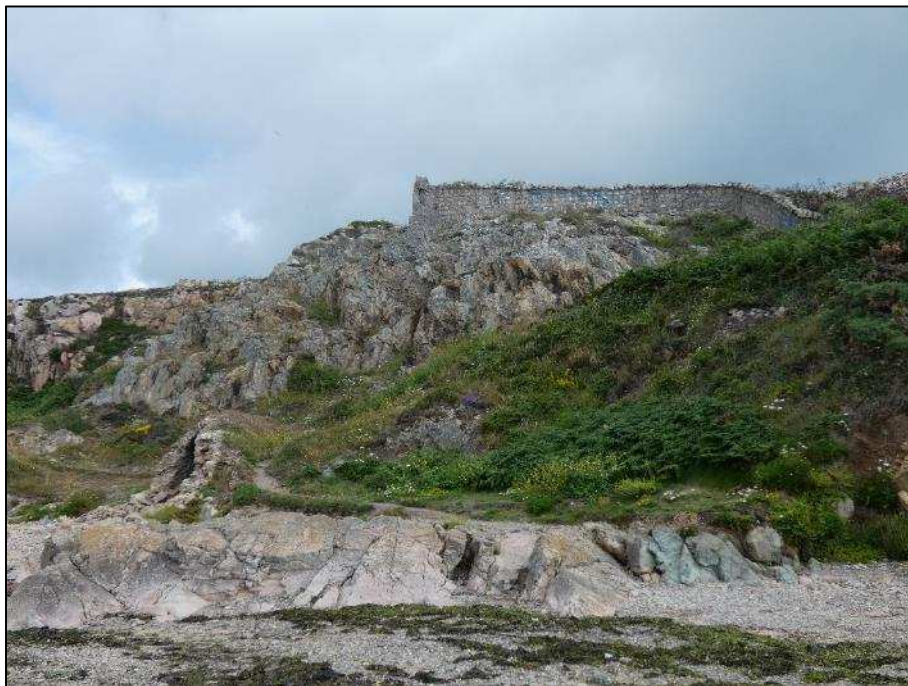
Plate 14. Coursed rubble granite wall with rubble granite coping and cement pointing
