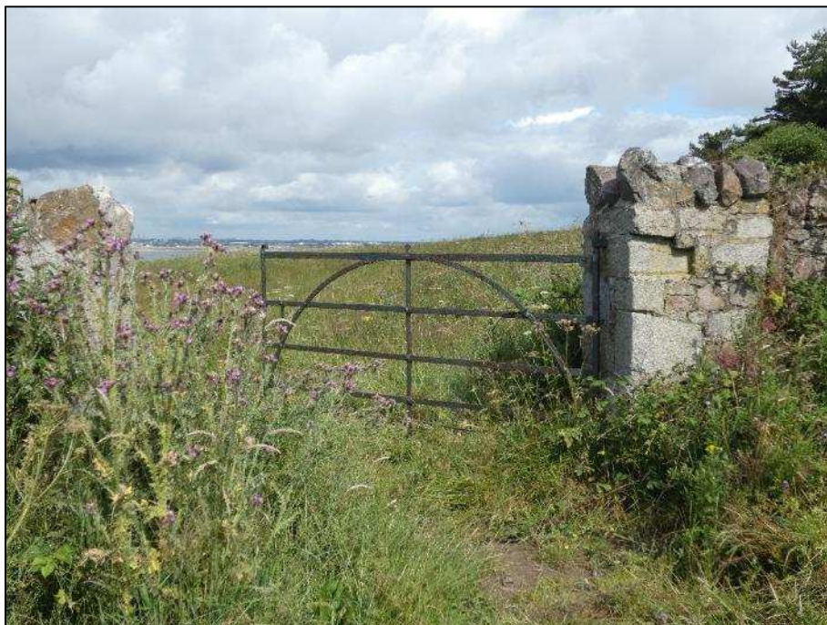
Plate 10. Wrought-iron gate supported on square profile gate piers with granite coping
