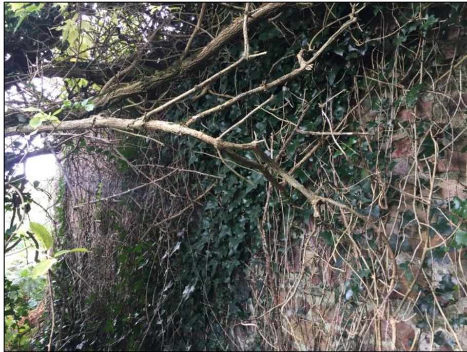
Plate 19. Quartzite boundary wall running east-west facing southeast
