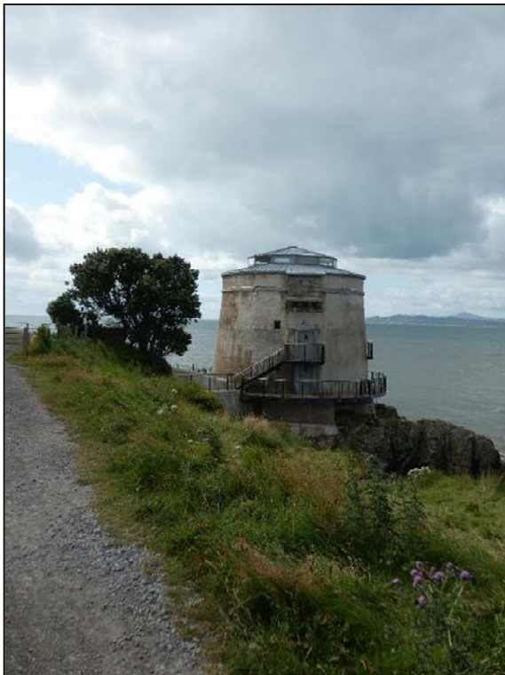
Plate 7. Martello Tower from north
