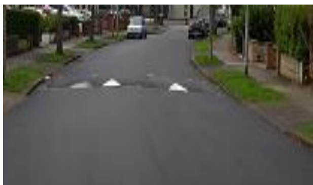
Newly installed Ramp - The Avenue, Rush, at St Catherine's National School
