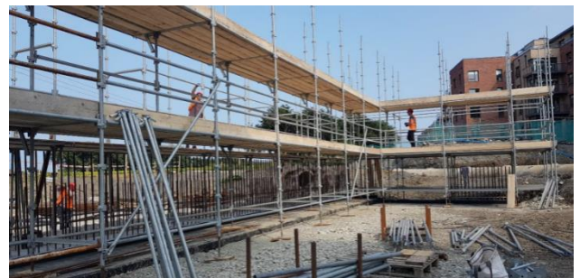
Scaffold erection for bridge southern abutment and wingwall
