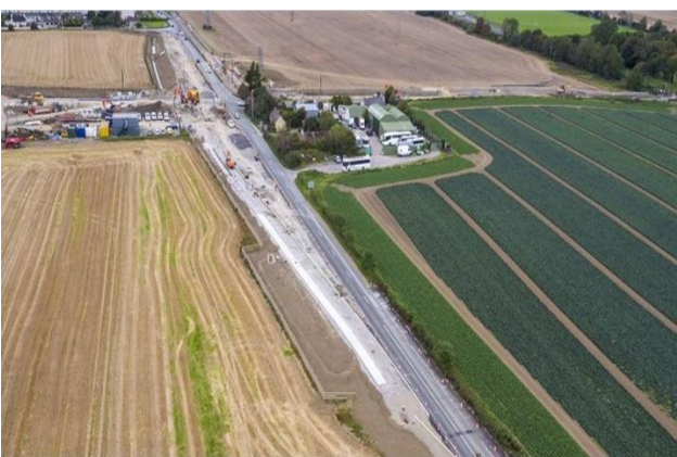
Looking westwards on Mayne Road – footpaths and kerbing being installed
