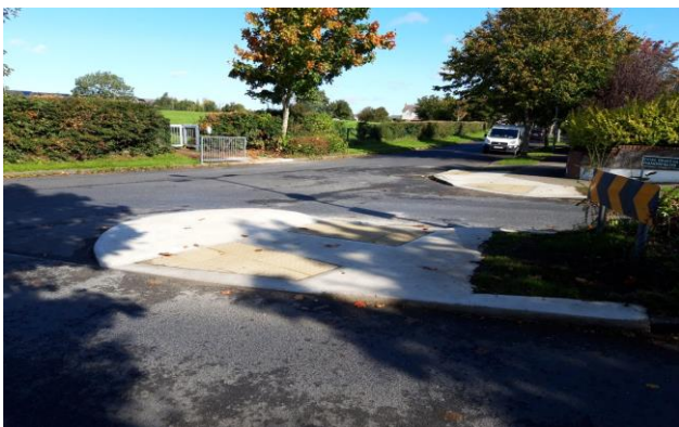
Newly installed footpath complete with tactile paving – Manorfields Avenue, Ongar
