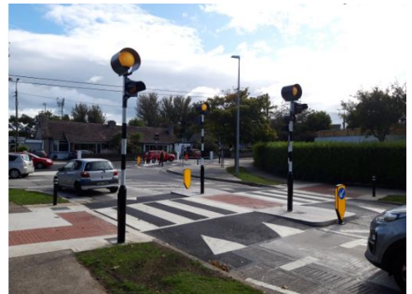
Barnageeragh & Dublin Road Junction Skerries altered to a roundabout with 3 raised Zebra Crossings on each arm.
