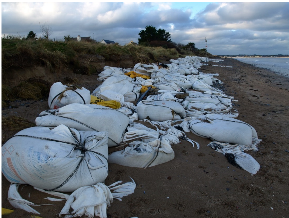
Figure 4-1 Private Landowners taking matters into their own hands in an attempt to protect their properties from coastal erosion.
