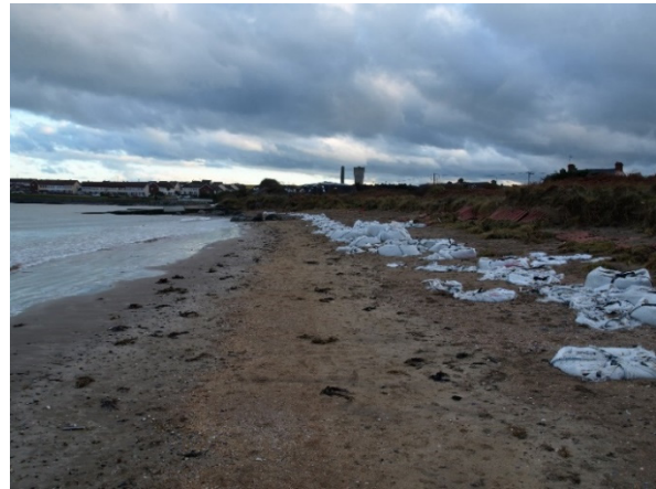
Figure 2-5 Sandbags put in place at Portrane by local residents to slow down erosion. Photo: Hans Visser
