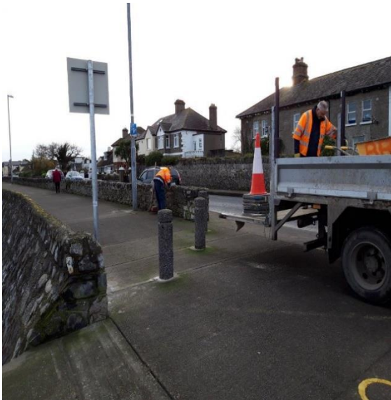
Installation of soft sand warning signs Baldoye Estuary
