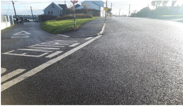
Upgrade of footpath near the new Crossing, Balbriggan Road, Skerries
