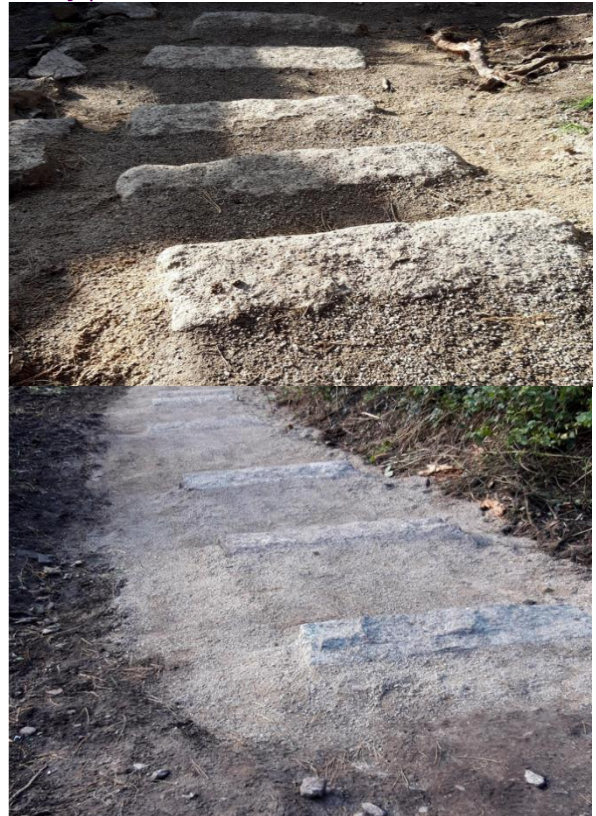
Restored steps and installation of 2 nd set of steps
