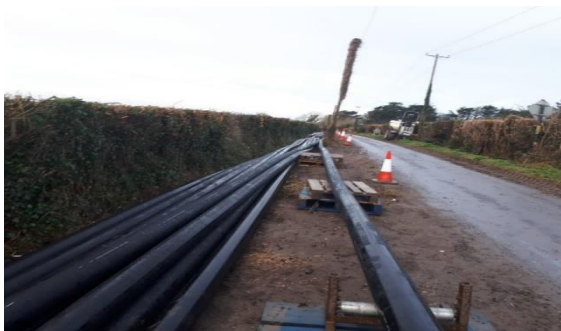
Loughshinny Foul Sewer Rising Mains progressing well.
