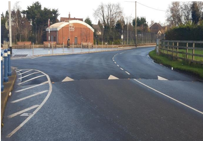
Newly installed Raised Table Ramp – Junction of Beaverstown Rd, Ballisk Ln & Main St, Donabate
