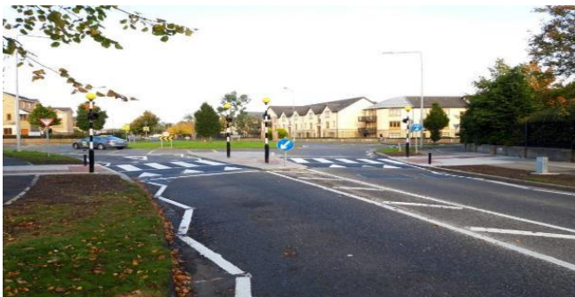
Diswellstown, Dublin 15 New Signalised Zebra Crossing which was Commissioned in December
