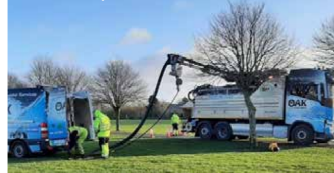
Specialist contractors on site at Ward River Valley Park
