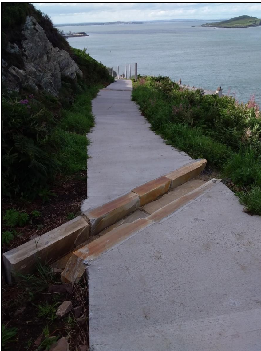
Plate 36 Perpendicular drains installed in concretised walking pathways.
