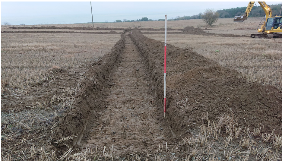
Plate 15: Trench 23 looking ENE
