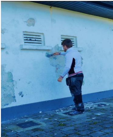
Community member in Rush painting the Rush Harbour toilet building October 2021
