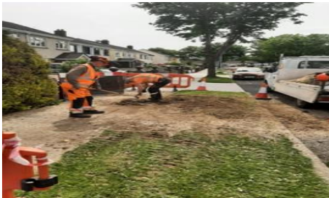
Stump Removal – Huntstown Green
