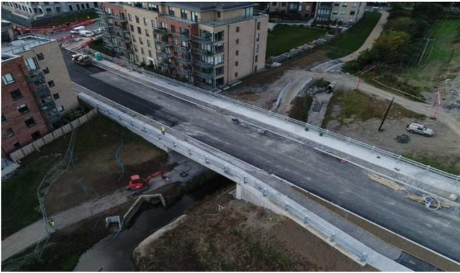
Aerial view of the new bridge and linear walkway under bridge
