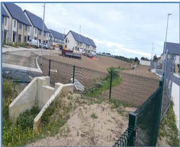
SuDS Device being construction in new Rush Development
