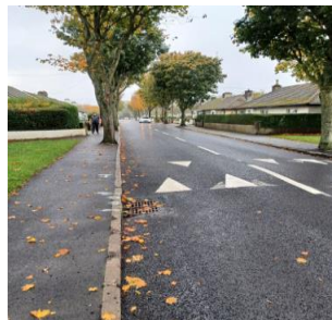
Road Resurfacing Works – Back Road, Malahide
