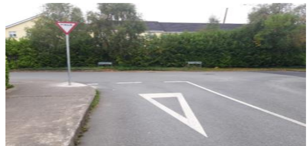
A Yield sign with associated line marking added St Mochtas Estate
