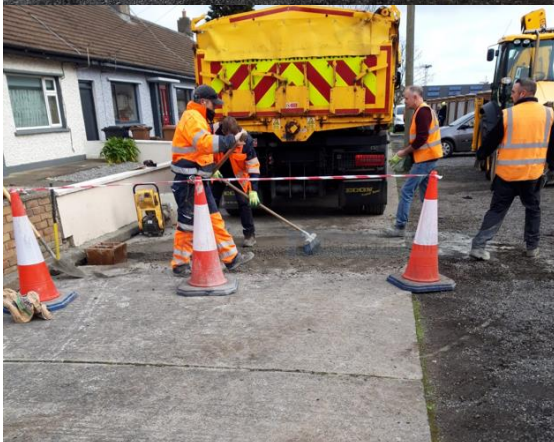
Church Road Howth - Pressure Washing of Granite Steps
