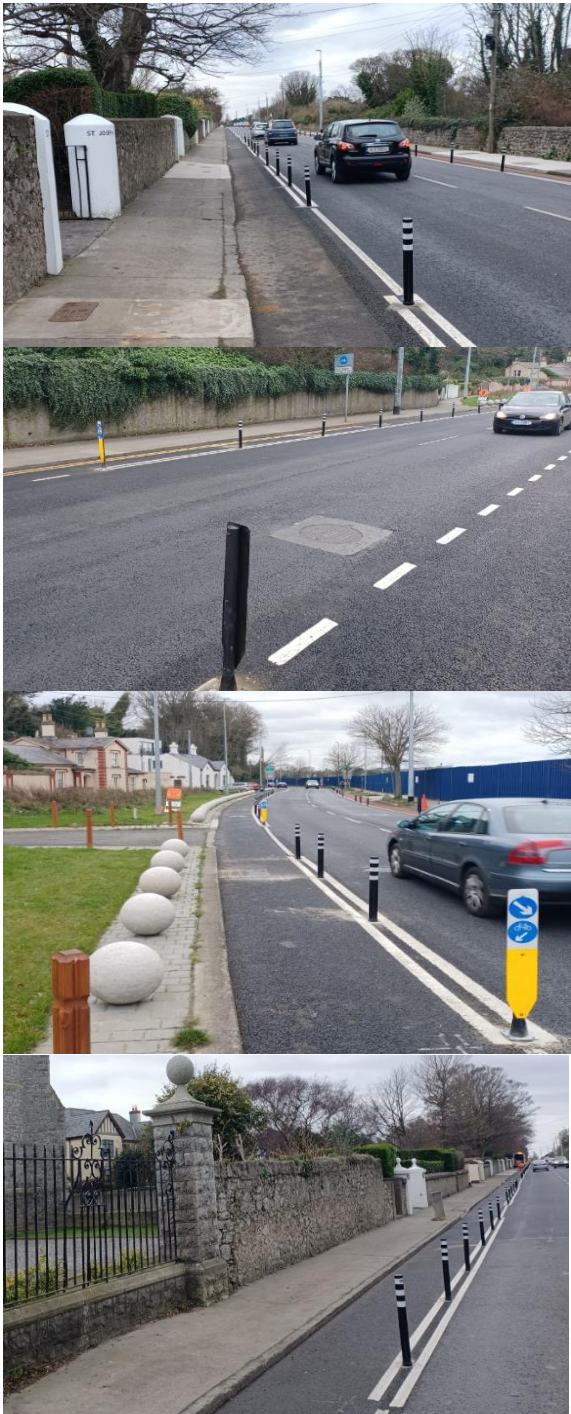
Baldoyle –Howth Protected Cycle Lane: Bollard install works on Howth Road
