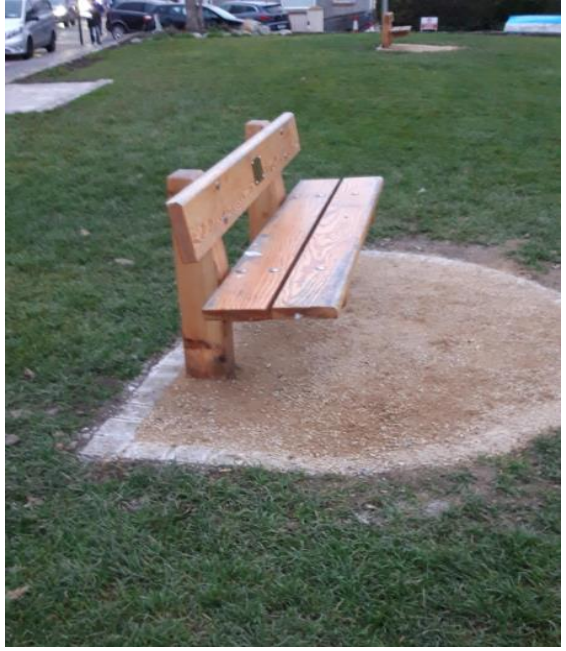
Resurfacing under existing seats
