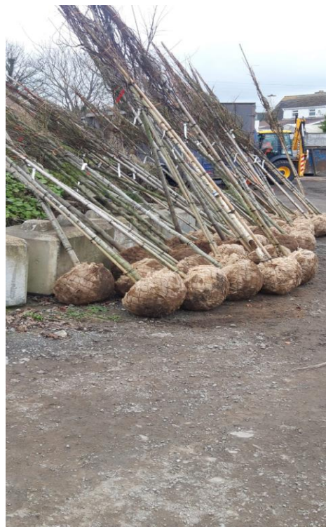
Delivery of Trees from Irish Nursery for planting in areas where trees were previously removed.
