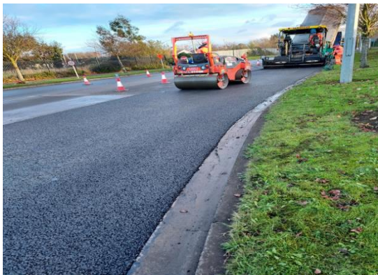
Castleknock Way and Crescent Surface Restoration
