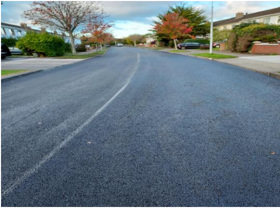
Ballycoolin Road Surface Restoration
