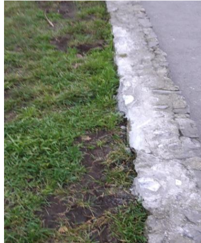
Before - The low limestone wall along the path edge has had the missing stones replaced and been repointed along its length
