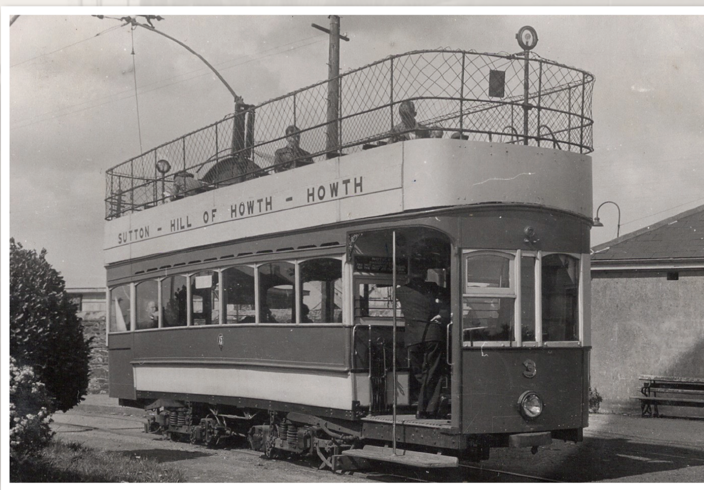
Hill of Howth Tramcar No.3 at Sutton Railway Station. Fingal Local Studies & Archives
