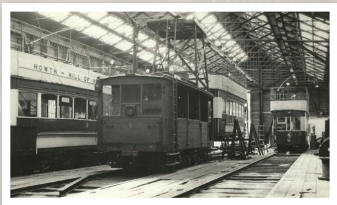
An interior view of the Sutton Carriage Shed showing Works Tramcar No.11 in the foreground. Fingal Local Studies & Archives
