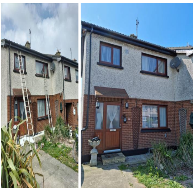
Recently painted dwelling pre/post works
