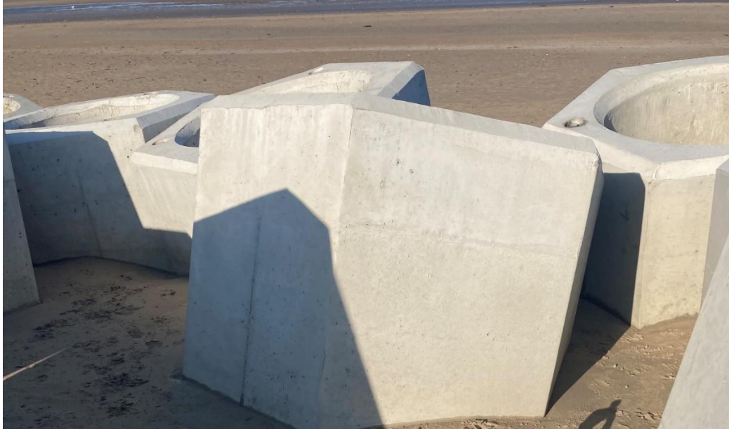
Figure 4. Coastal erosion structures found on Portrane beach.
