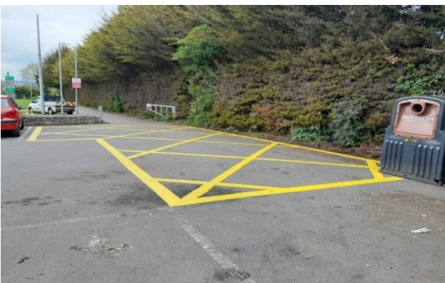
Porterstown Car Park - Relining of Yellow Box
