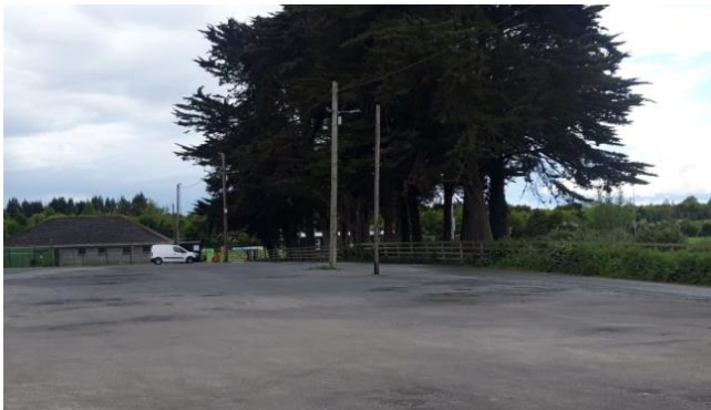
Installation of lights adjacent to the ESB poles at the car park in Ballymastone, Donabate
