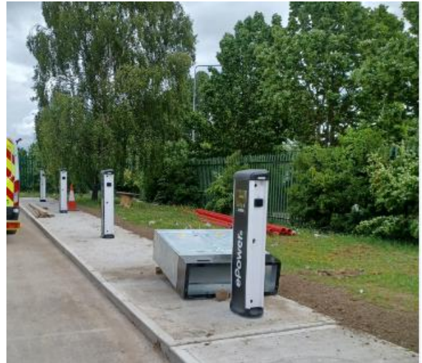
Watery Lane Depot EV charging hub gets underway
