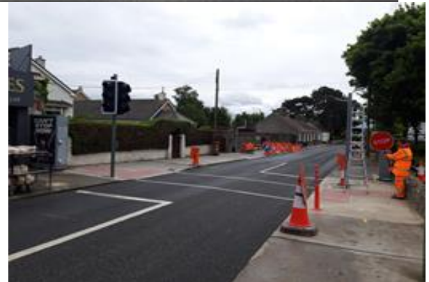
Signals upgrade underway between the Hill Top stores –R124-Malahide
