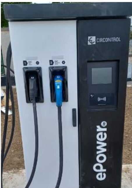
First 50KW DC charger installation goes ahead in Watery Lane
