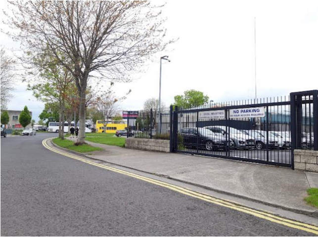
Double yellow lines installed on Porters Avenue in Coolmine Industrial Estate
