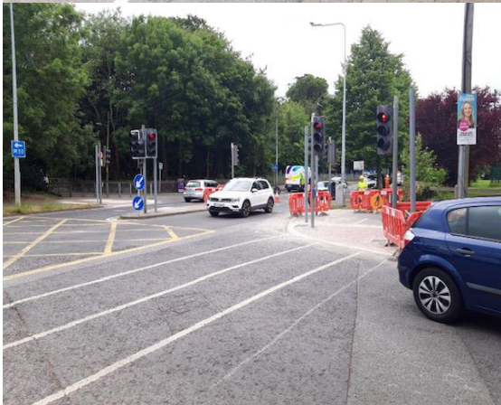
Junction of Snugborough Road and Grove Road upgrade works in progress
