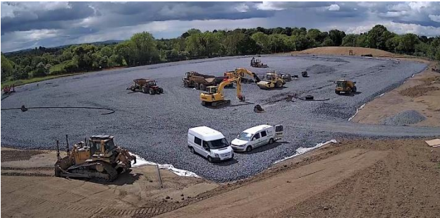
View looking southwest taken shortly after completion of stone base layer
