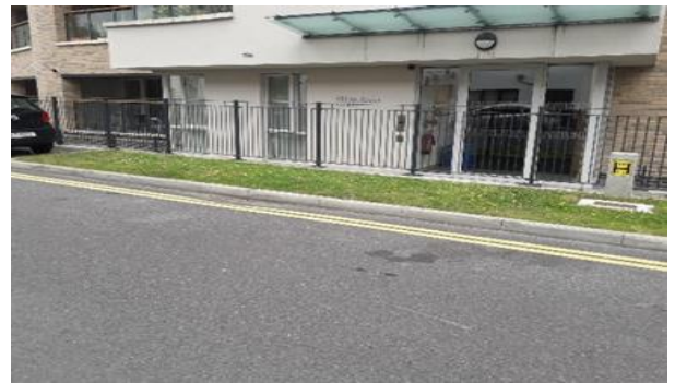
New Road double yellow lining in Red Arches-Silverbanks to improve visibility exiting underground residential carpark
