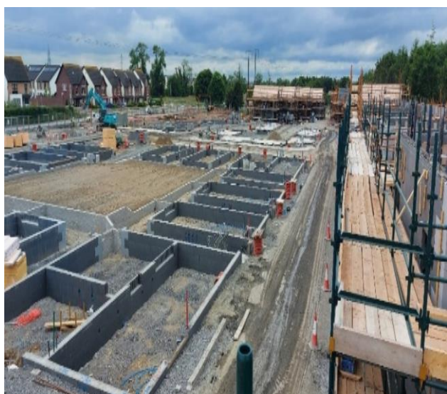
New houses being built in Hollystown using Insulated concrete formwork (ICF)
