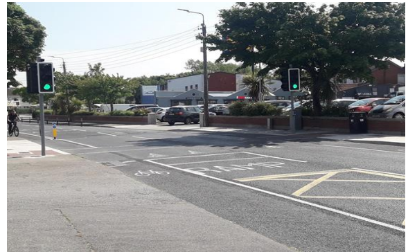
Civil works and Signals upgrade completed on Grange Road by Lidl entrance (used as a school warden crossing also)
