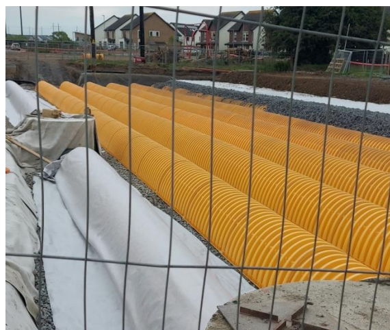
A new sustainable urban drainage system (SUDS) being installed in Hollystown.
