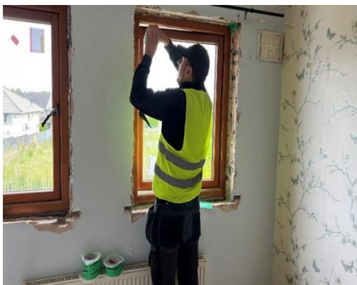
Window replacement in Jugback Estate.
