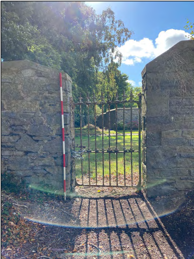
Plate 16: Gateway leading from graveyard to Glebe House, facing east-southeast.
