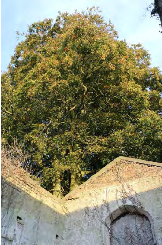
Figure 5: Western crown above eastern gable end of church.
