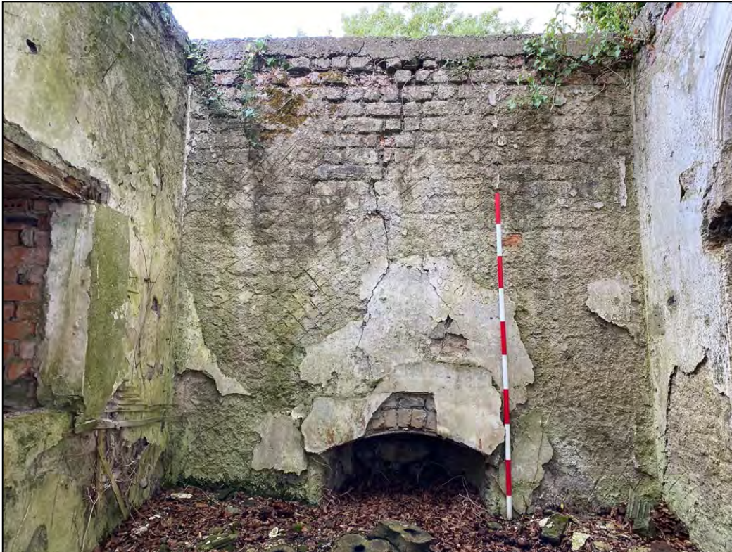
Plate 9: View of fireplace in vestry, facing northeast.
