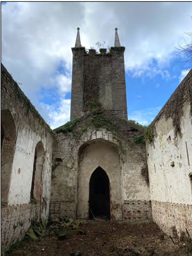
Plate 6: Interior of church with nave and bell tower, facing west-northwest.
