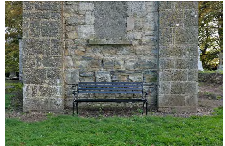
PIC. 20; RECENTLY-INSTALLED SEAT AT BASE OF TOWER..
