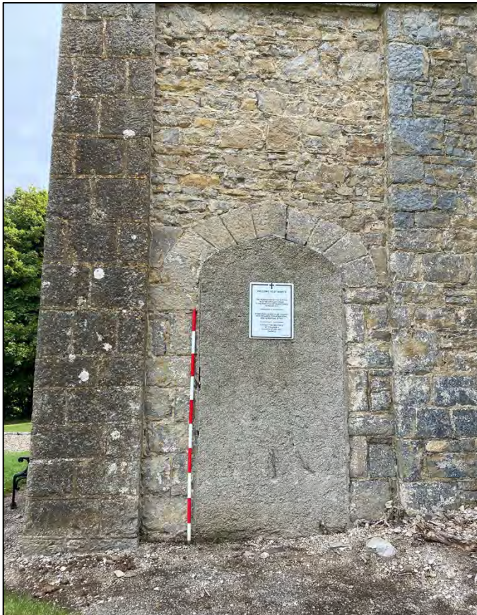
Plate 12: Blocked-up church entrance via bell tower, facing north-northeast.
