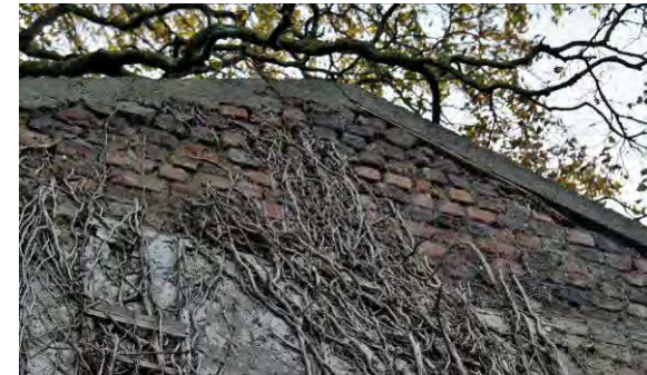
PIC.8; TOP OF EAST GABLE.
