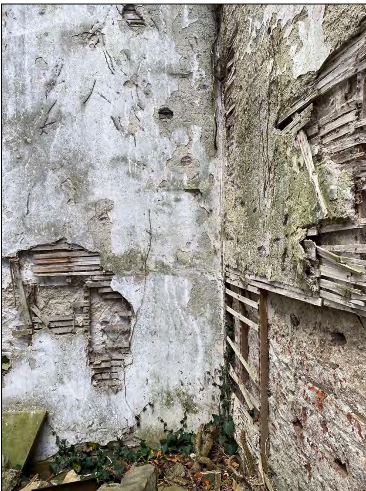
Plate 10: Timber wainscot panelling and extant render in southwest corner of nave.
