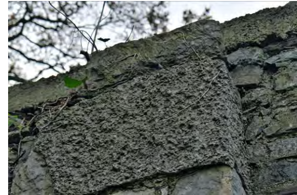
PIC.13; CONCRETE TOPPING TO STONE WALLS.
