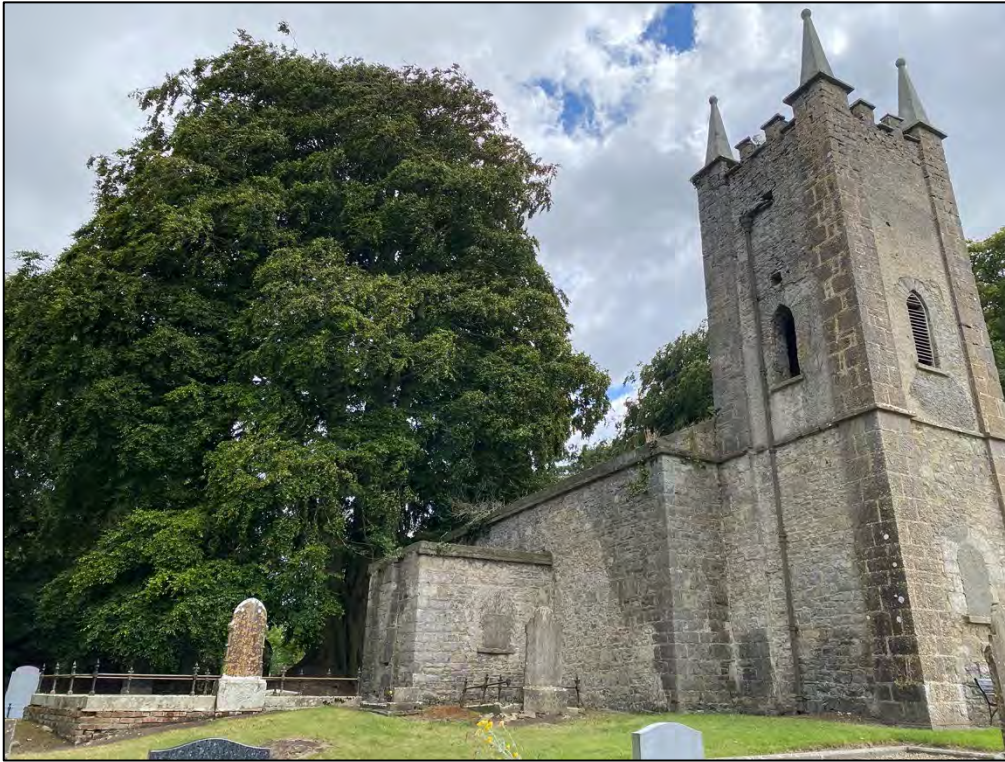
Plate 1: View of St Mary's Church, facing east-northeast.
