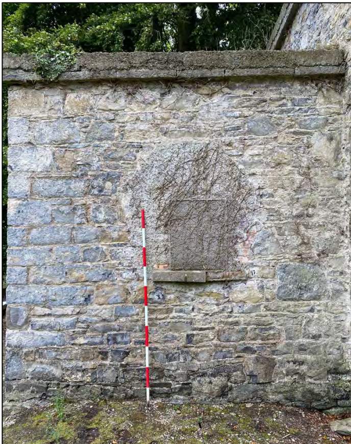
Plate 14: Blocked-up window in vestry, facing east-southeast.
