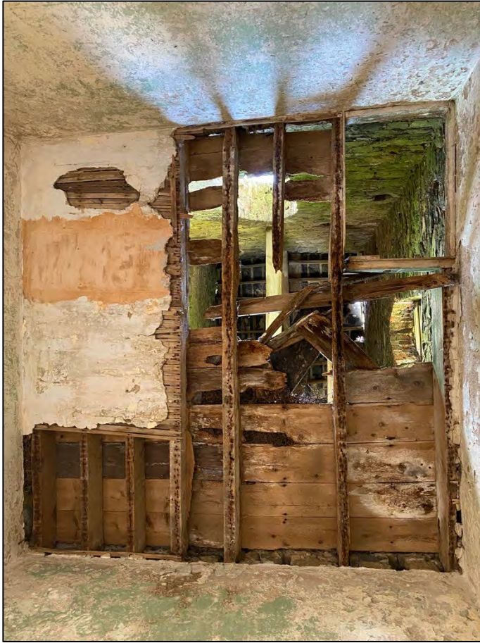
Plate 11: First level timber flooring in bell tower.
