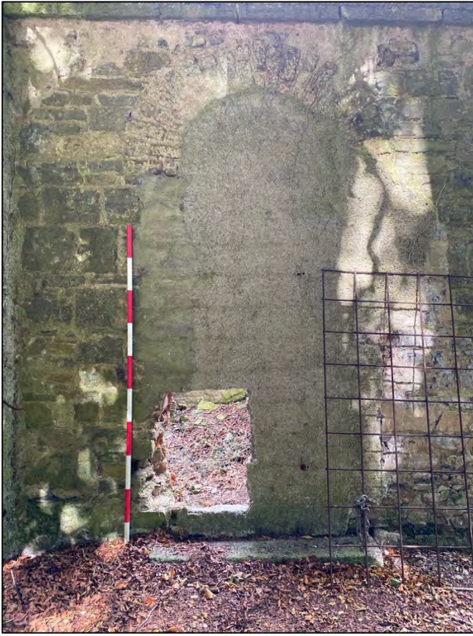
Plate 13: Blocked-up church vestry entrance, facing west-northwest.
