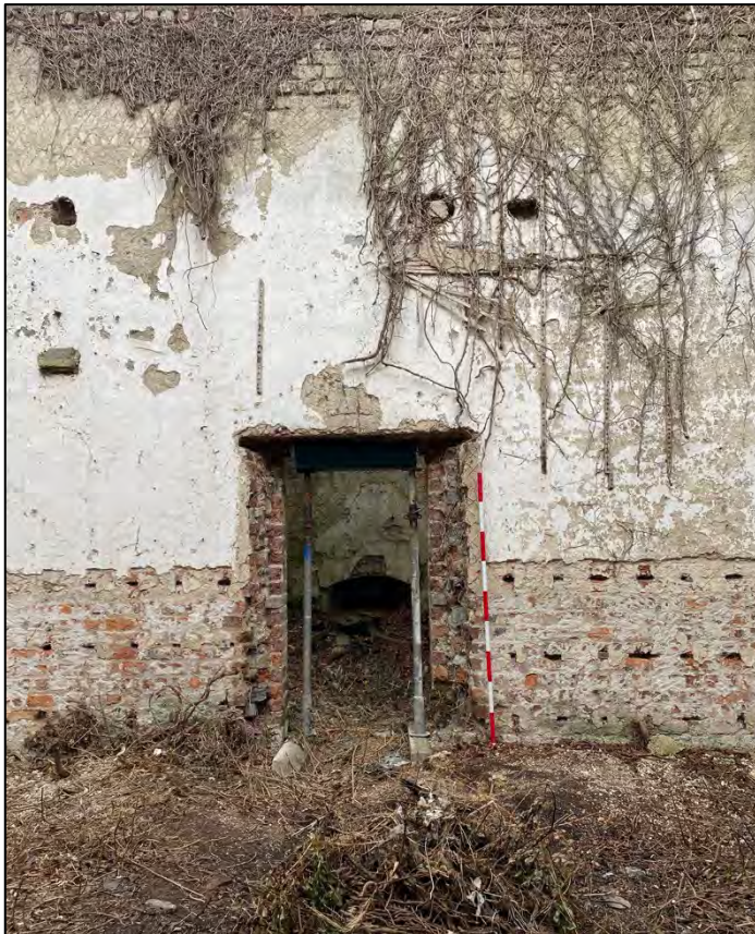
Plate 8: View northeast from nave to vestry, note propping of door.
