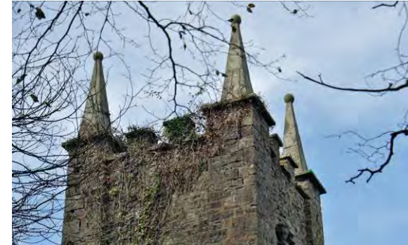
PIC.7; TOP OF TOWER.
