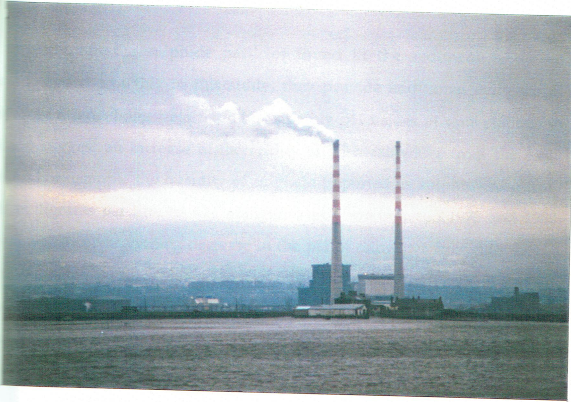
Figure 4.11 : The twin ESB cooling towers at Poolbeg in Dublin Port are one of the most significant sources of SCP's. This generating station replaced the Pigeon House power station in 1967.
