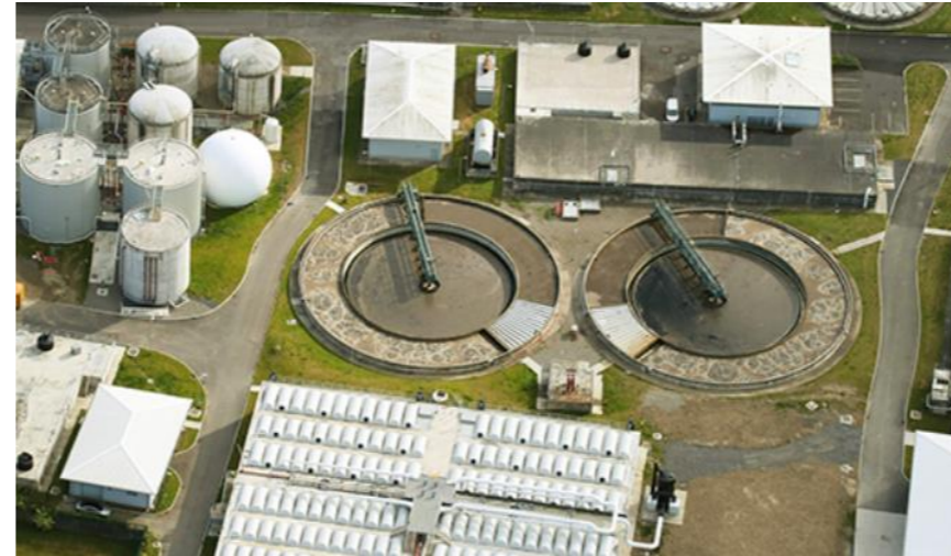
Figure 9-1: Swords Wastewater Treatment Plant
