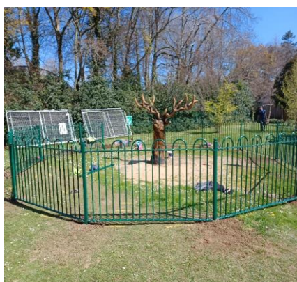
Fence erected and looking well.
