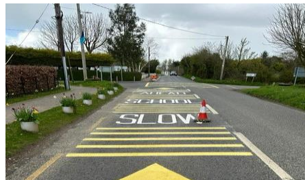
Garristown National School - School Road Markings
