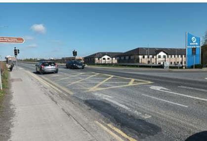
Above: New School Markings for Scoil an Duinigh (Riasc centre entrance) and Yellow Box for Feltrim Road junction/Riasc Centre
