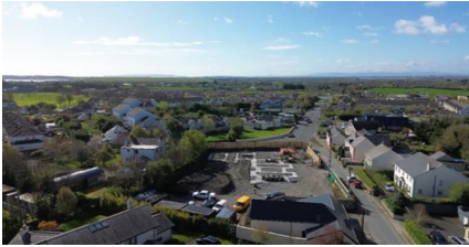
Fingal County Council - construction scheme at Ballough Place, Lusk – 10 dwellings
