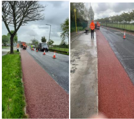
Images of red SMA cycle paths being installed along Brackenstown Road.
