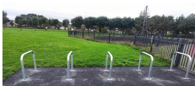
Recently installed Bicycle Stands at Racecourse Park Playground, Baldoyle, Co. Dublin
