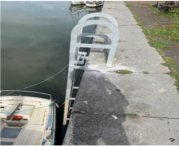
New Steel Access Ladders East Pier
