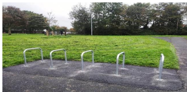
Recently installed Bicycle Stands at Seagrang Basketball Court, Baldoyle, Co. Dublin
