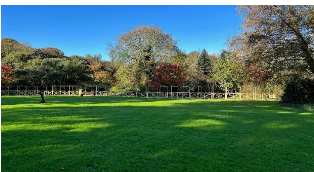
New light feature under construction, West Lawn, Talbot Botanical Gardens.
