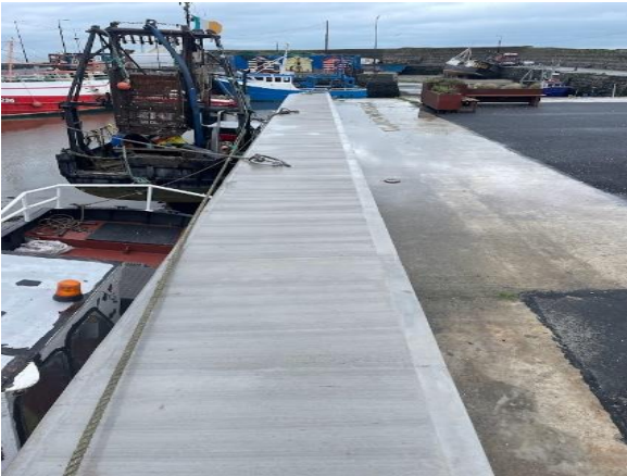
Concrete Plinth with Mooring Bollards East Pier
