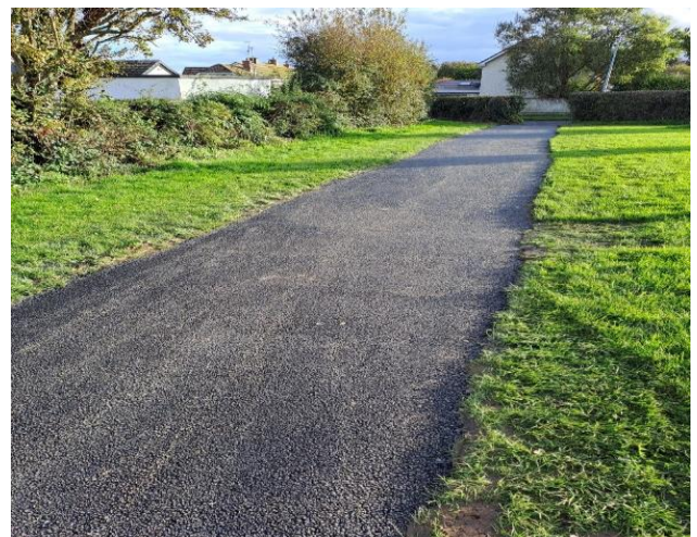
Newly installed paths across the open space at Tara Court Balbriggan.
