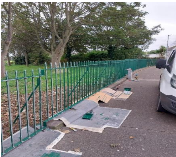
Refurbishment works to park railings at Seagrang Drive.
