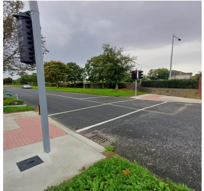
A new pedestrian crossing was added on Lohunda Road to existing traffic lights
