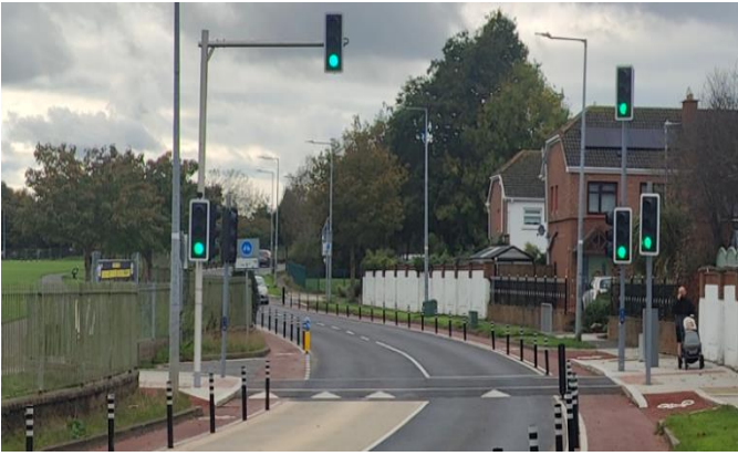
Brackenstown Road, Swords - New Toucan Crossing - collaboration between Active Travel and Traffic Operations.
