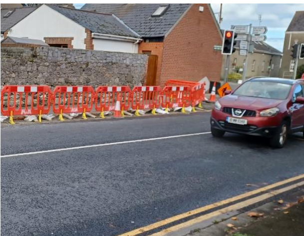
Willie Nolan Road – Footpath Upgrade works
