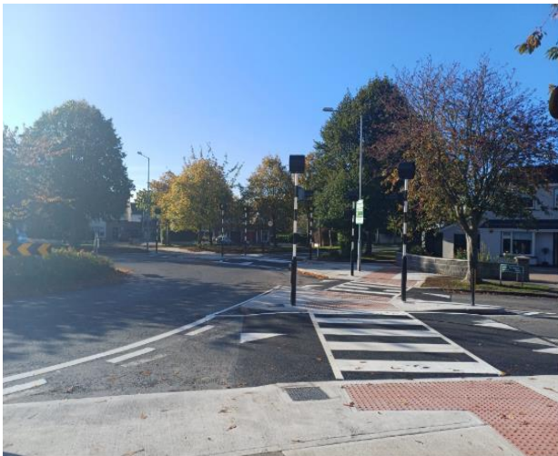
New four-arm raised zebra crossings on Carpenterstown Avenue/Laurel Lodge Road
