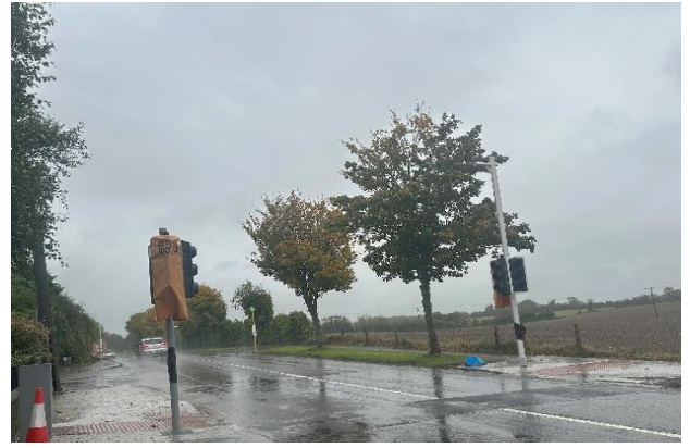
Dublin Road, Lusk - New signaled pedestrian crossing in progress.
