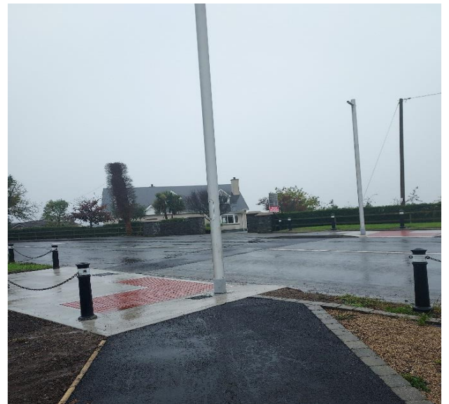
Loughshinny- New signaled pedestrian crossing in progress.
