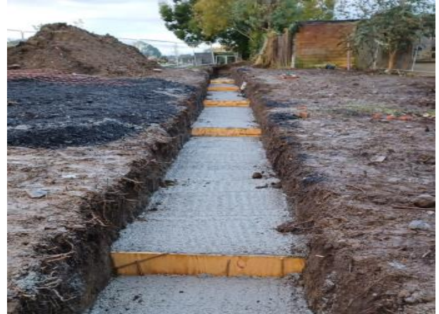
Laying of boundary wall foundations at Balgriffin cemetery
