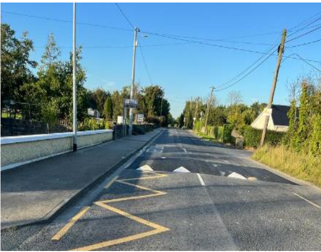
Kilcoskan National School - The Ward, Co. Dublin - New Traffic Calming Speed Ramps
