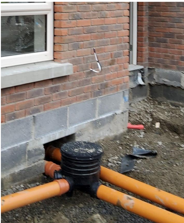
Checking Drainage in houses in Clonsilla.
