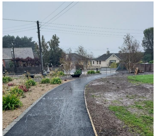
Loughshinny- New pathway connecting new signaled pedestrian crossing to the village.
