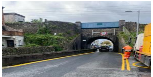
Claremont Road-Howth Road Junction - New STOP sign and STOP Markings and refreshing existing road markings by Railway bridge-Strand Road below
