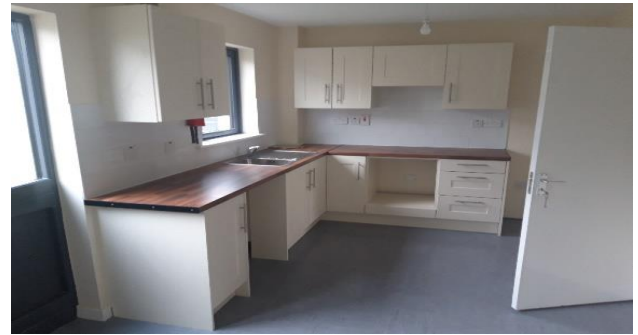
Kitchen/Bathroom refurbishments in Dublin 15
