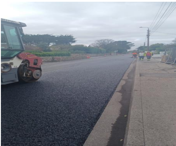
2023 POW Greenfield Road Inlay
