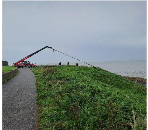
Martello Balbriggan wreck removed by the Operations Department
