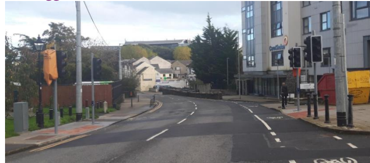
Bridge Street, Swords - New Toucan Crossing - awaiting ESB connection.
