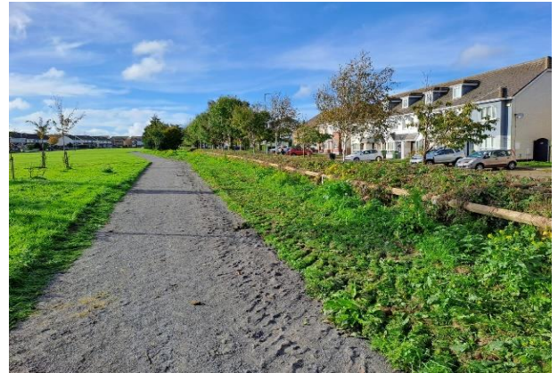
Newly constructed pedestrian pathway between Westbrook and Moylaragh Estates Balbriggan
