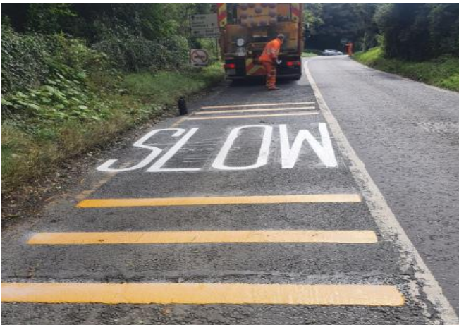
Swords area - Crossroads at Brackenstown Road and R108 - Emphasised SLOW road markings on approaches.
