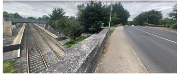
Figure 1 - View from Rail Bridge towards Granard Bridge and Blanchardstown
