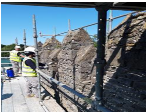
Knights and Squires Wall Consolidation and Repair
