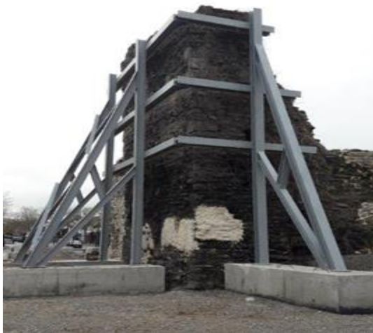
East Tower - Temporary Bracing
