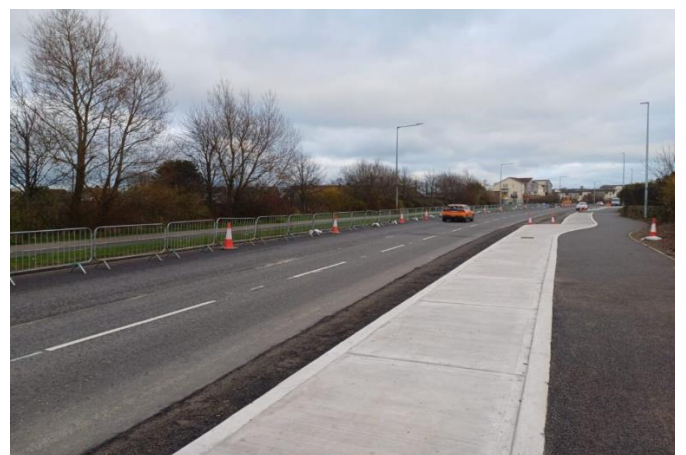
Works completed on the south side of the Hamilton Road
