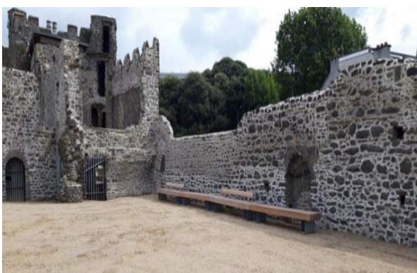
Knights and Squires Chamber and Wall After Repair
