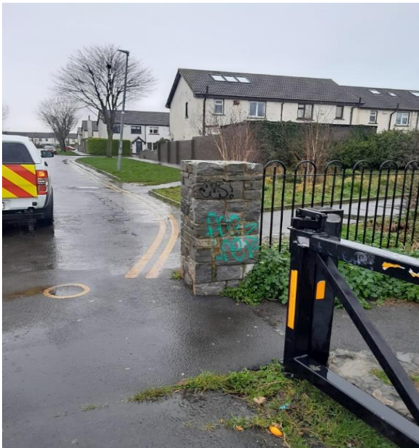
Graffiti removal Red Arches and Seagrang Baldoye completed.
