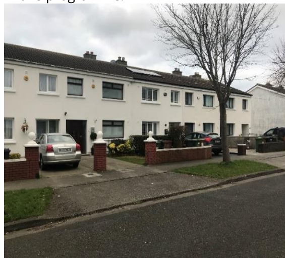
Post-works – Strandmill Estate, Portmarnock (external wall insulation, new windows and doors)
