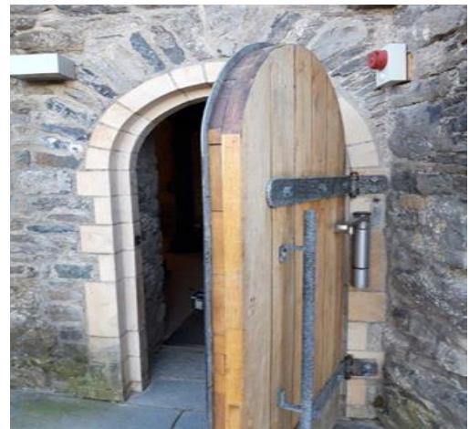
Chapel Door - Before and After Alteration
