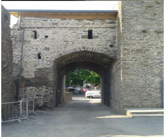
Gate House - During and after Works
