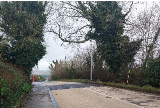
Naul - New Traffic Calming Ramps in the proximity of Naul National School
