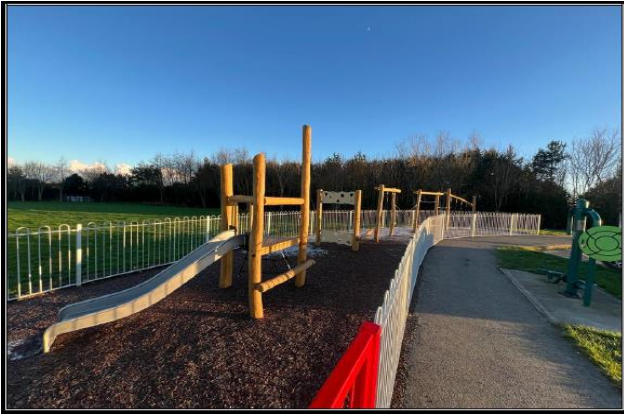
Pictured above, Kettles Park Trim Trail installed and completed.
