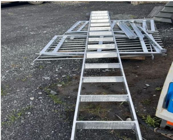
Replacement ladder for High Rock, Malahide due to be installed at location once weather and sea conditions allow.
