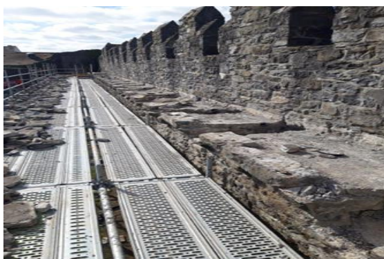
Wall Walk Being Installed
