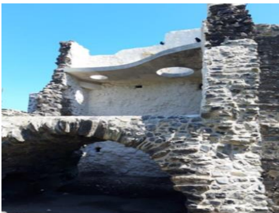
East Tower External and Internal Views after Consolidation and Repair
