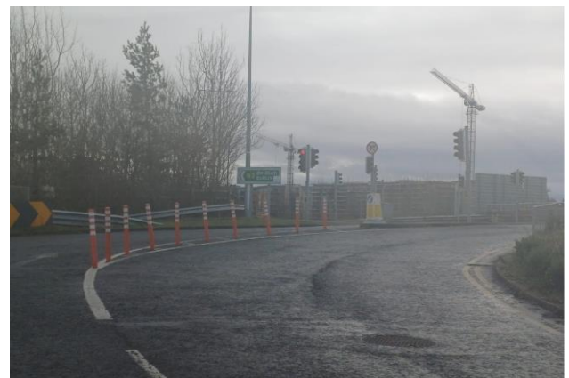
Flexible bollards are placed exiting Navan Parkway to delineate traffic entering and exiting the train station.
