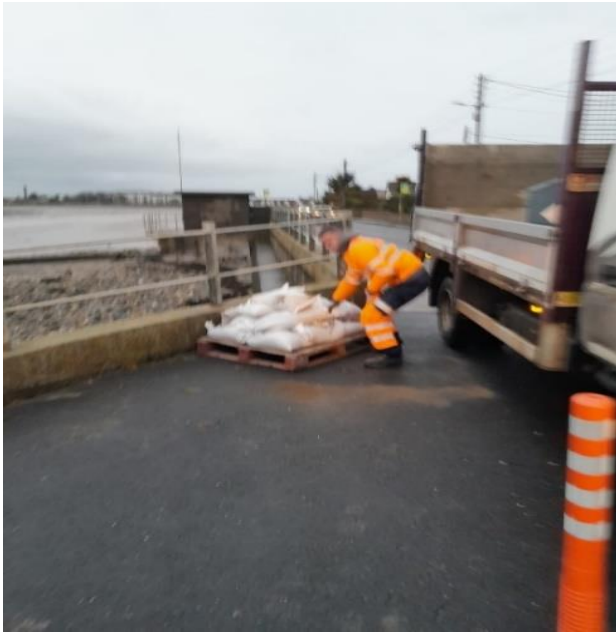
Sand bag delivery at Sutton Strand due to threat of sea overtopping. There was no breach at high tide.
