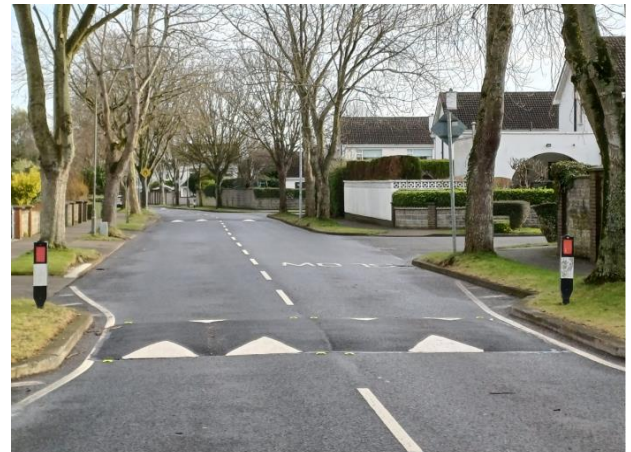
Traffic calming ramps on Delwood Road completed with permanent paint and reflectors.
