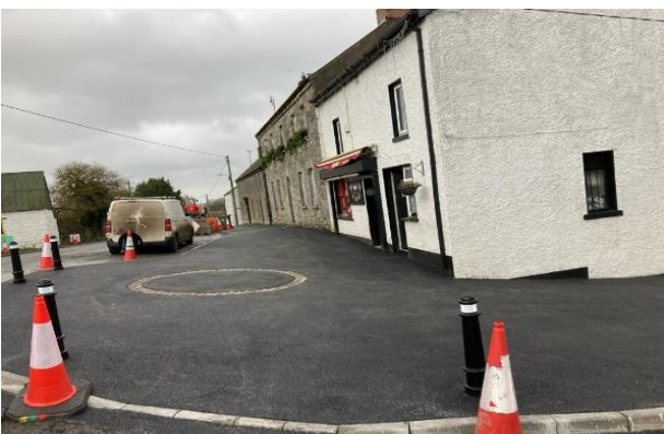
Garristown- New Kerb Build Out Garristown Main Street
