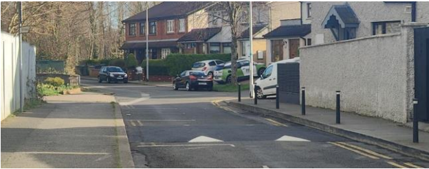
Swords – Chapel Lane - Speed Ramp Replacement
