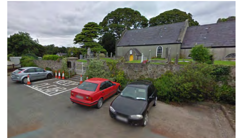
Fig. 8-14: View of Parking at the Square
