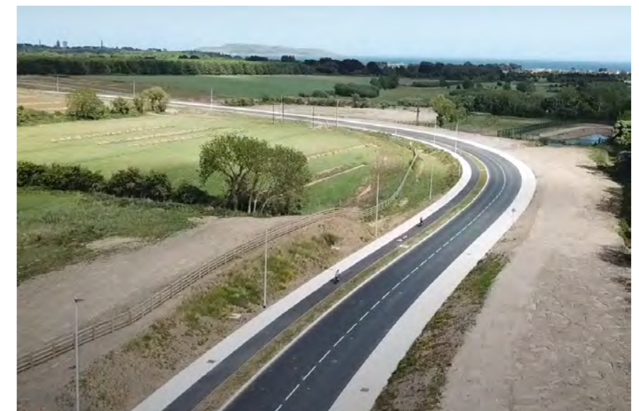
Fig. 1-4: View of Donabate Distributor Road
